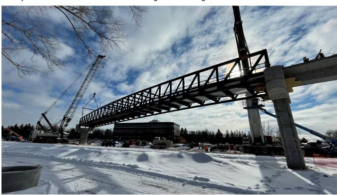
Crews placed the bridge span for the Beltline Boulevard regional trail bridge over the freight rail tracks this past week. Watch a time-lapse video of crews setting the span.
