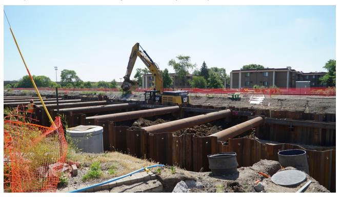
With one half of the Blake Regional Trail underpass constructed on the west, crews are working to build the eastern half. Sheeting has been installed to support the excavation activities. Once excavation activities are complete, crews will advance tunnel construction.
