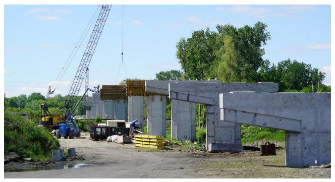
As LRT travels into Hopkins a bridge structure is needed for LRT to cross over freight rail tracks, as seen in the background of this image. The piers for the LRT bridge continue to take shape.
