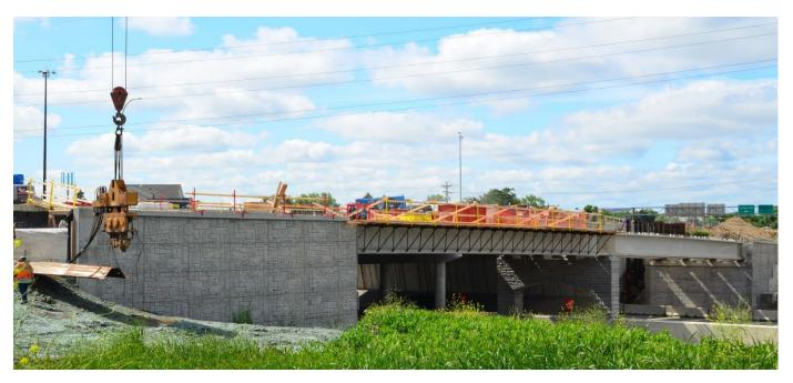
With beams already set-in place crews are advancing bridge deck construction for the I-494 Bridge at Flying Cloud Drive in Eden Prairie. Crews build forms in the daytime while the majority of concrete is poured at night during a road closure.
