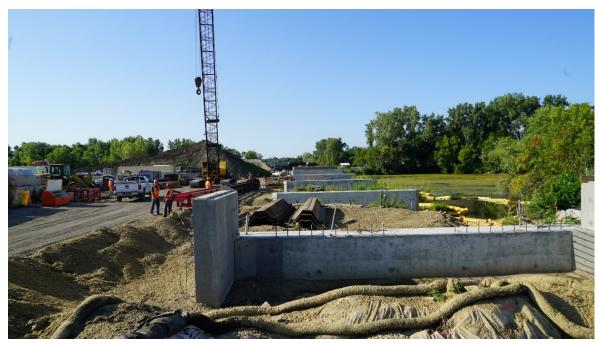
The Minnetonka-Hopkins LRT bridge is located east of Nolan Drive and west of the Hopkins Landfill. The bridge piers are emerging near K-Tel Drive. Excavation and piling for the bridge piers will move south towards Smetana Road. The bridge will carry the LRT vehicles over the freight tracks in the very background of the photo.
