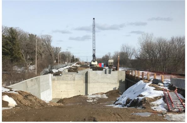
The abutments for the freight and trail bridge over Minnehaha Creek are complete, with bridge deck work and backfill coming this spring.
