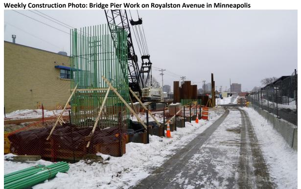
Progress is being made on the LRT bridge spanning from Royalston Avenue over North 5<sup>th</sup> Avenue and North 7<sup>th</sup> Street. Crews are working on the bridge piers and abutments, with intermitent pile driving in the area.
