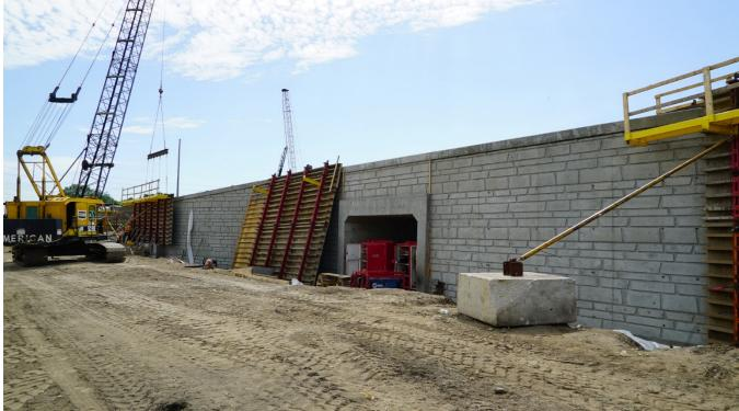
The pedestrian underpass will provide access under freight rail for residents and visitors traveling to destinations north of the station area. Crews are completing the concrete work for the tunnel.
