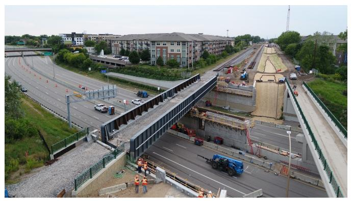
The freight railroad bridge is just starting to be pulled off of its old abutments and shifted to its new permanent location. Moving the bridge took a fraction of the time intended due to its excellent design and advanced construction planning. Watch the full bridge move here.
