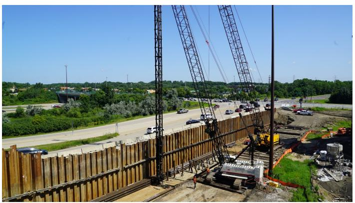
Crews are installing sheet pile and associated infrastructure to support the future LRT tracks. Significant amount of sheeting for the SouthWest Station has been completed. Crews will transition to working on the bridge structure crossing Technology Drive and Prairie Center Drive.
