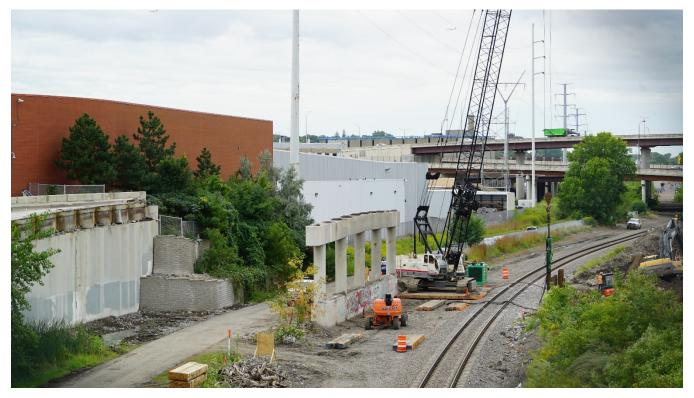
The old Glenwood bridge is almost fully demolished. Crews removed the deck and girders that once spanned the rail corridor and bike trail. Work on retaining walls, bridge abutments and piers continues in the area. Work activities are coordinated with active freight traffic.
