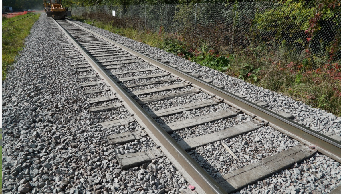
New Freight Rail Track
