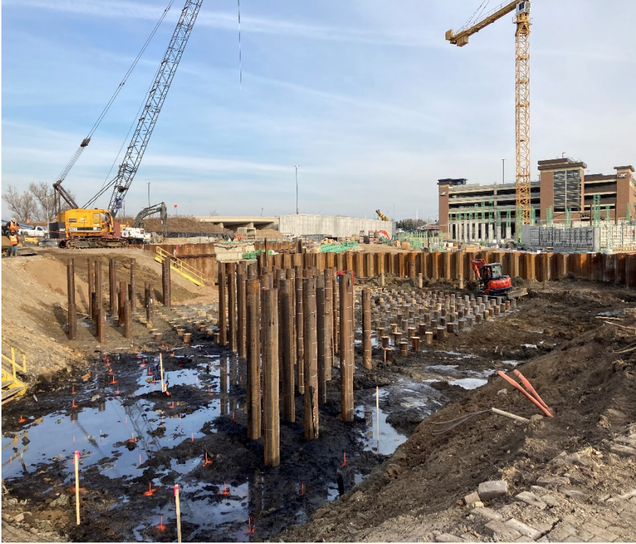
Looking east: pile supports for bus loop
