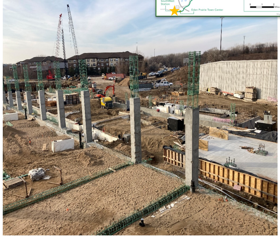
Looking west: construction of station waiting area and track foundation
