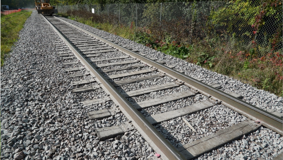
New Freight Rail Track
