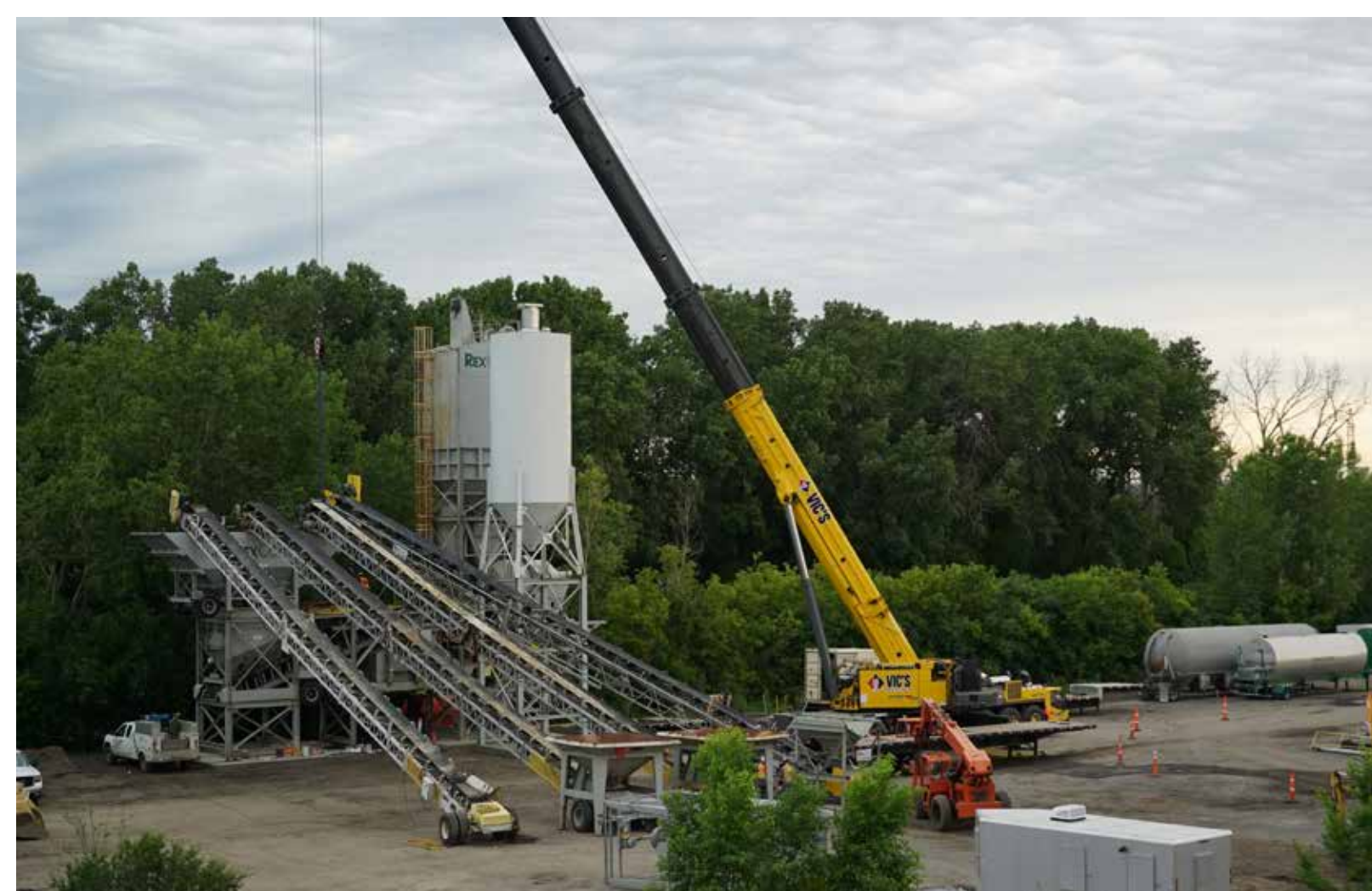
Establishing a concrete batch plant in Linden Yards
