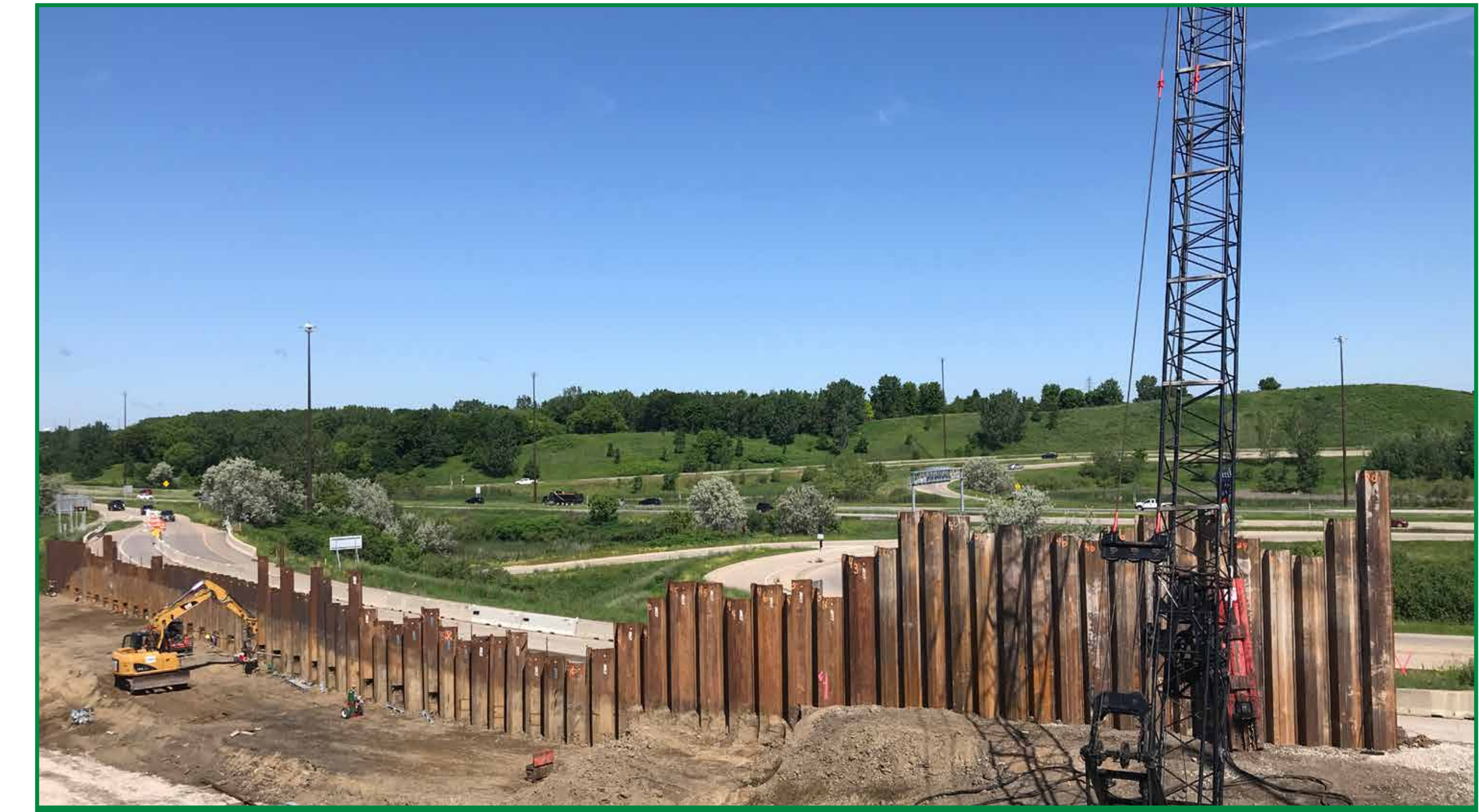
SouthWest Station Area Retaining Wall Underway
