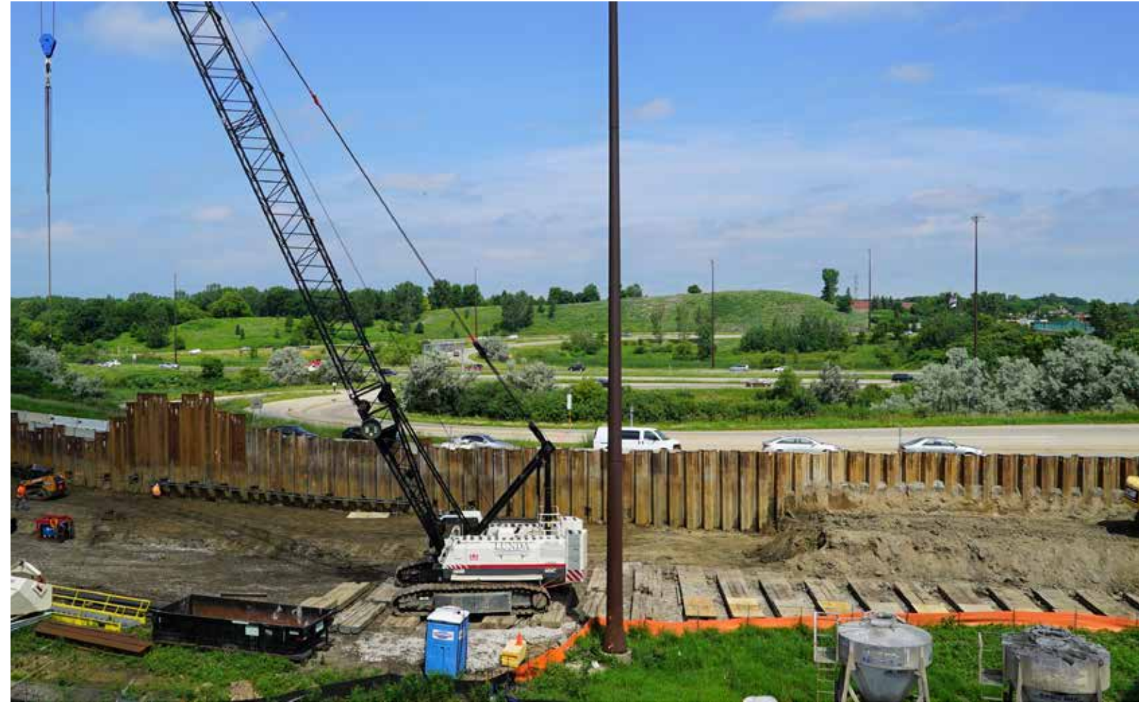
Retaining wall work at SouthWest Station
