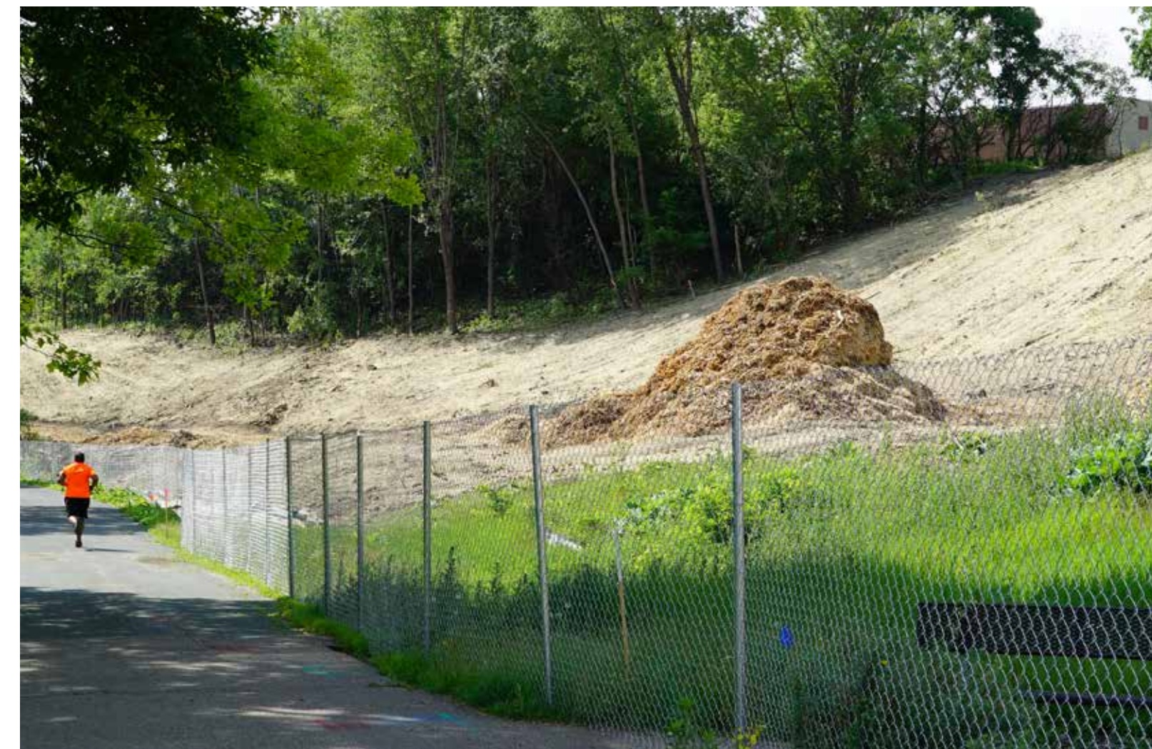
Earthwork for site preparation
