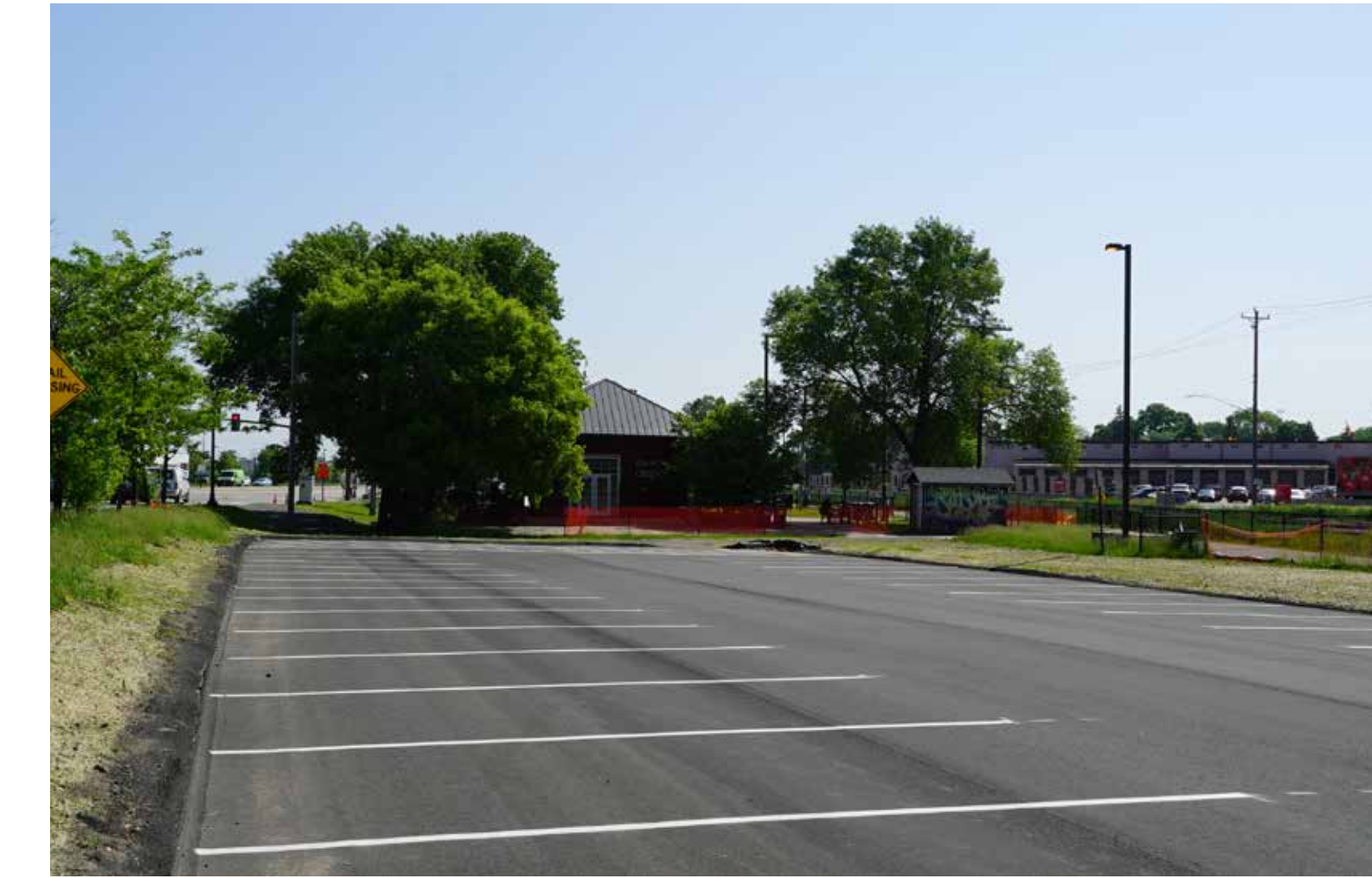
Temporary Hopkins Depot Parking lot to accommodate Excelsior Bridge Construction
