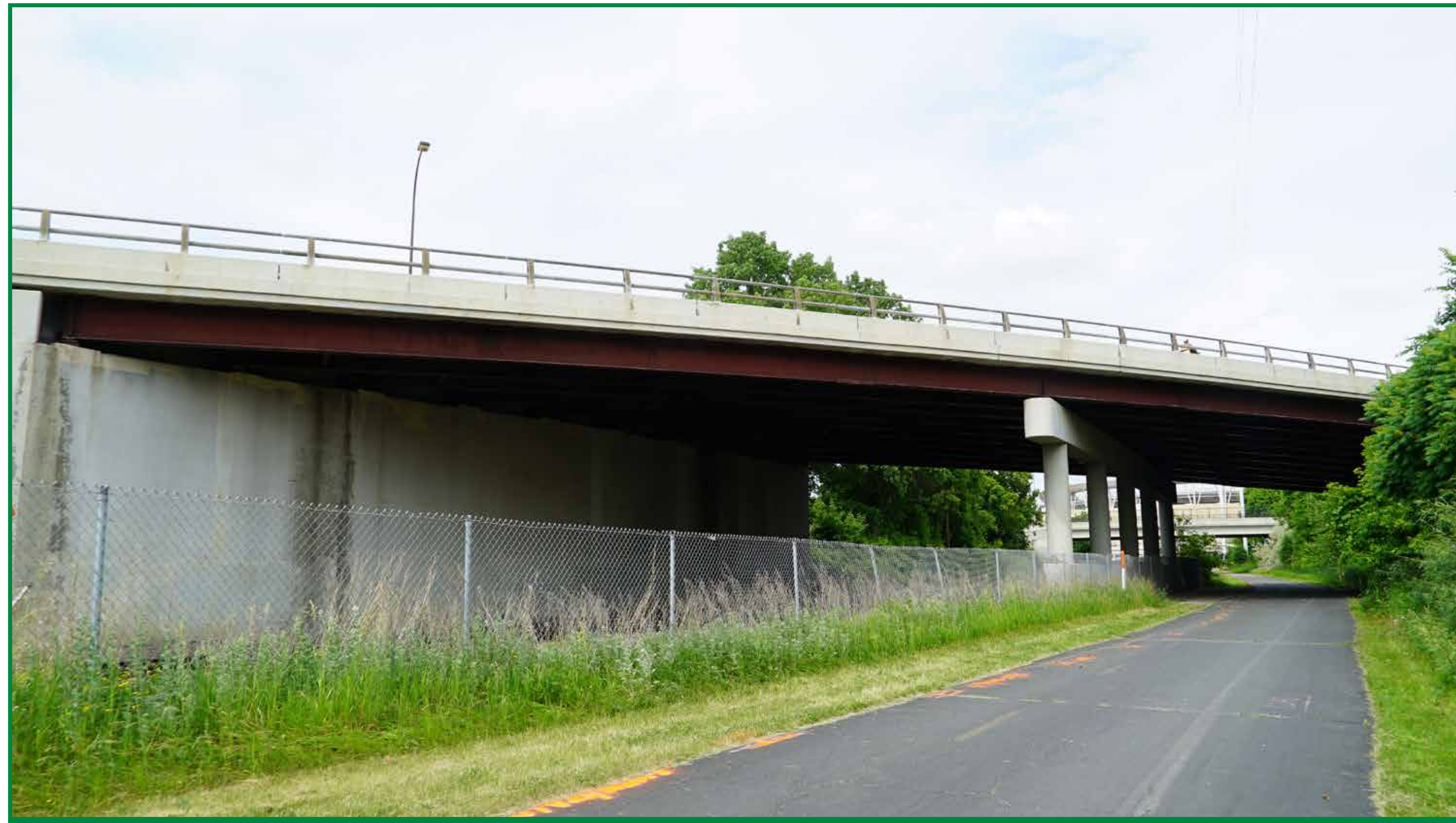
Glenwood Avenue Bridge Pre-demolition
