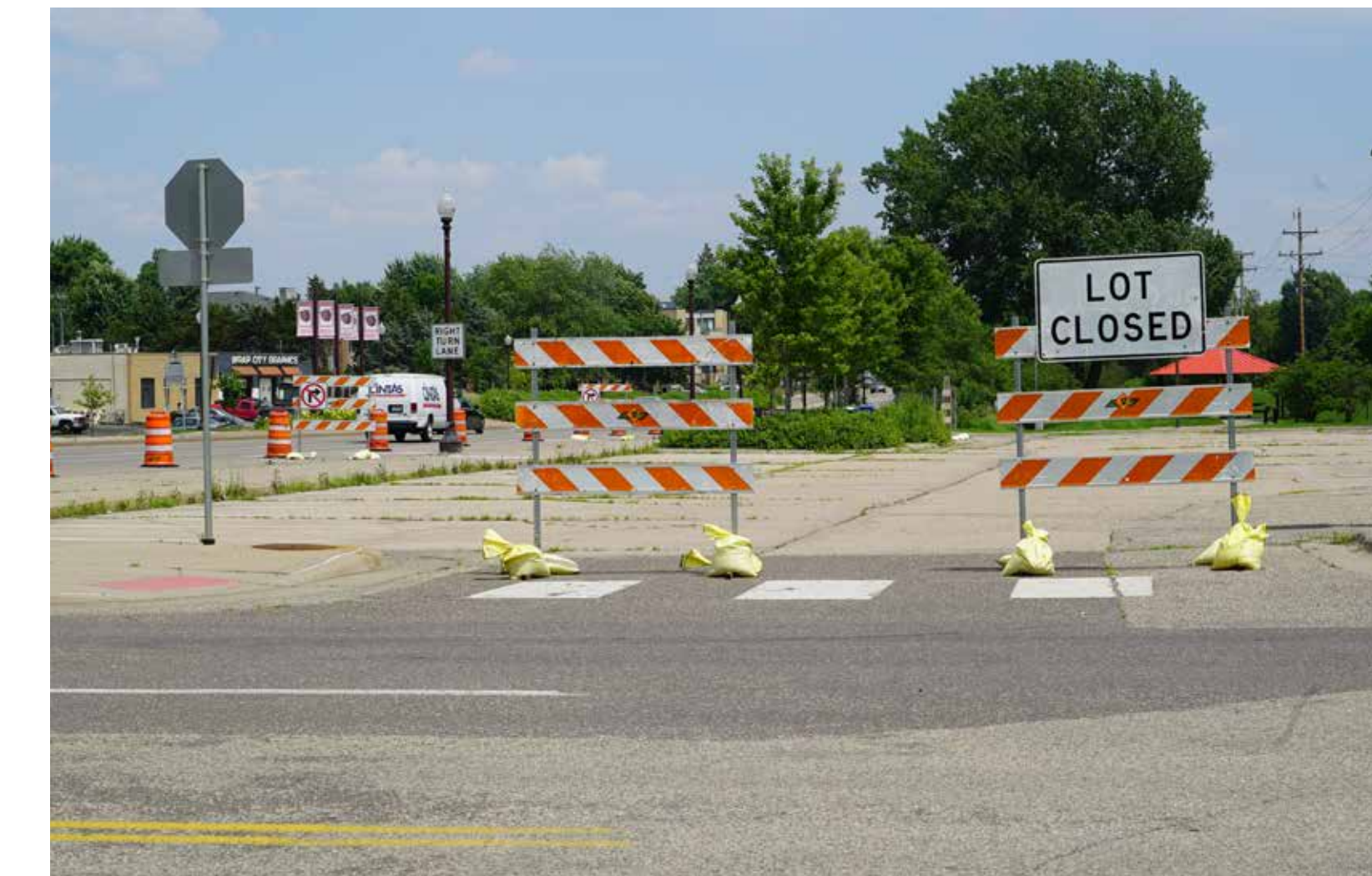
Work between 5th Avenue and 8th Avenue
