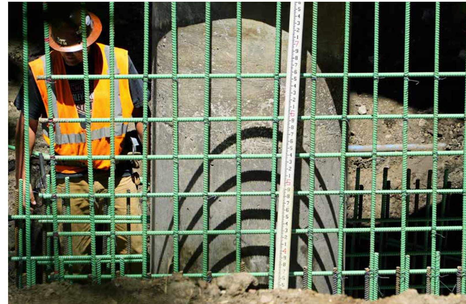
Pier protection work at I-394
