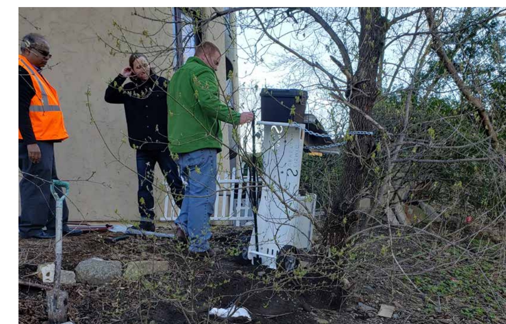
Vibration monitoring in sensitive locations
