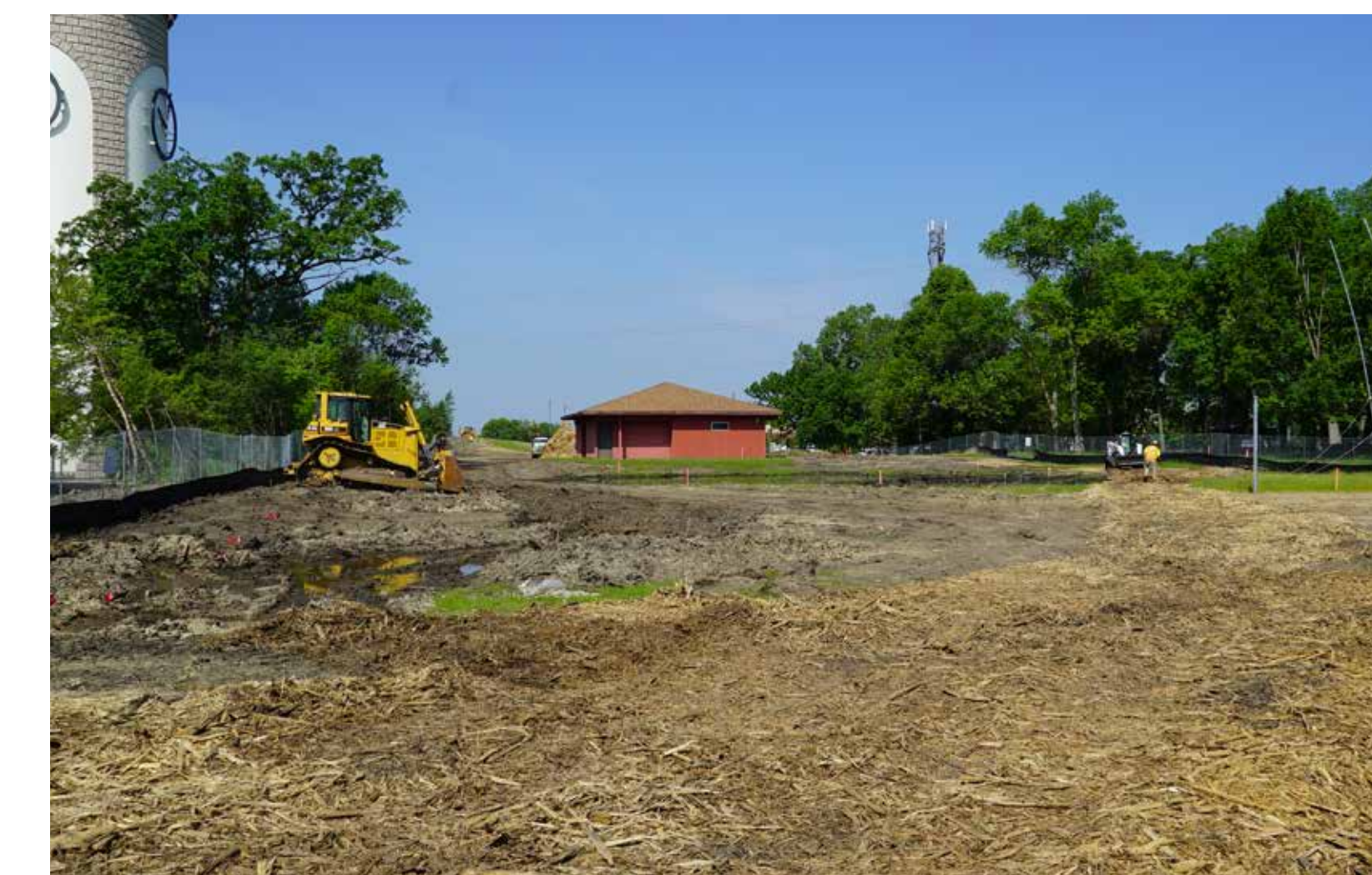
Clearing and grubbing
