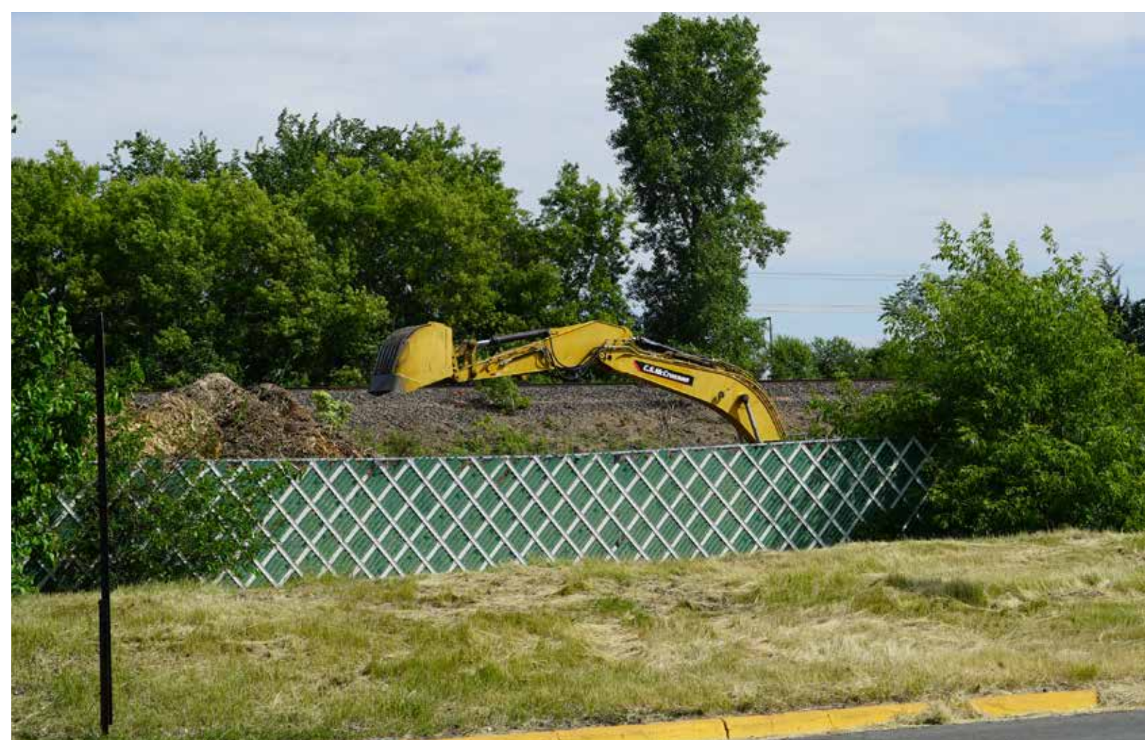
Building access ramp to corridor
