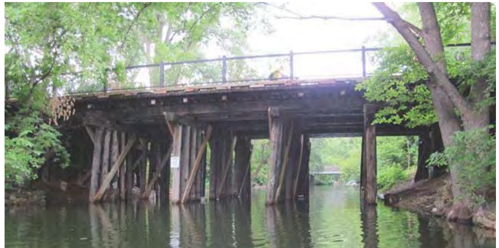
Old Cedar Channel Freight Rail Bridge
