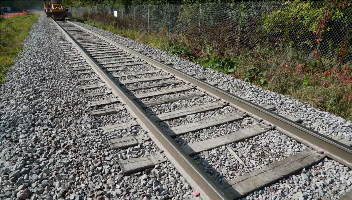
New Freight Rail Track
