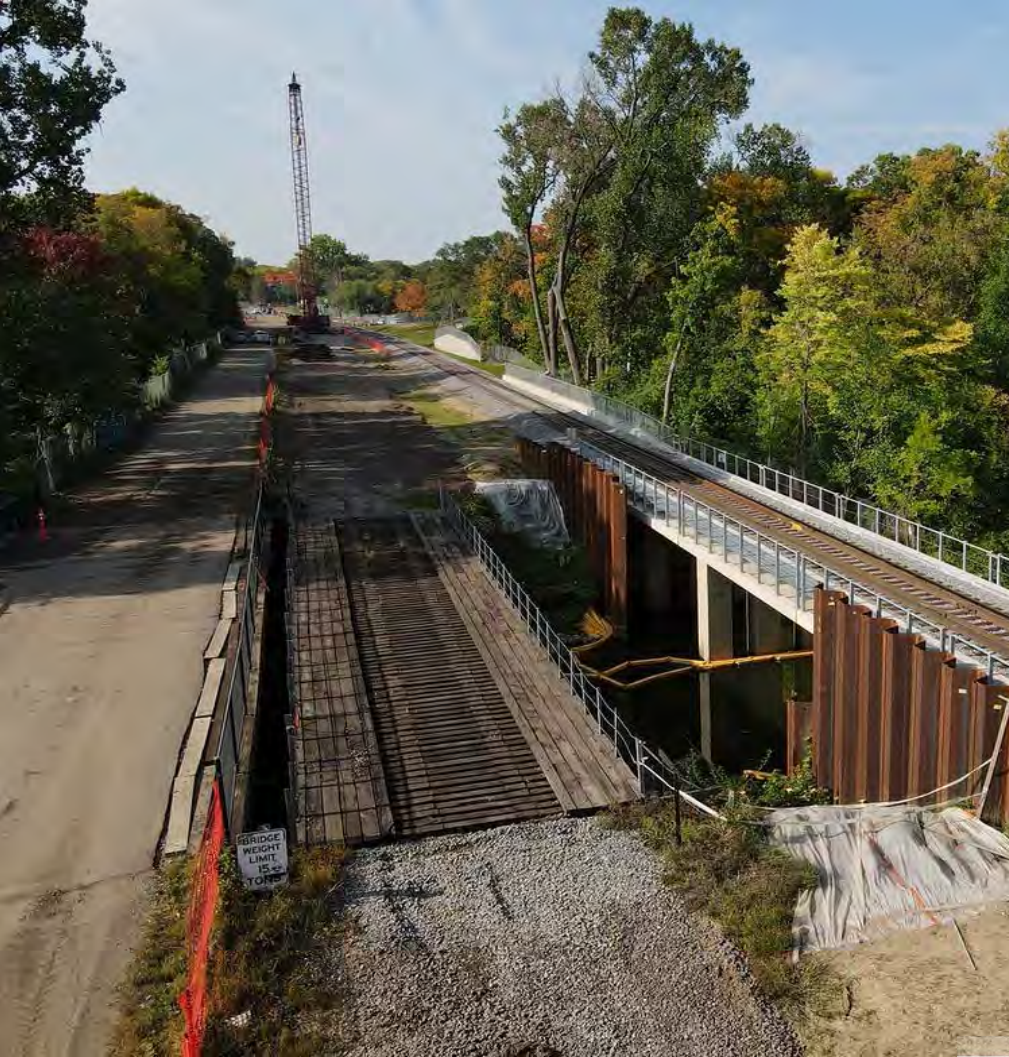
Old Freight Rail Bridge
