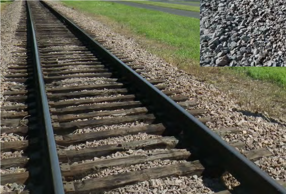
Old Freight Rail Track
