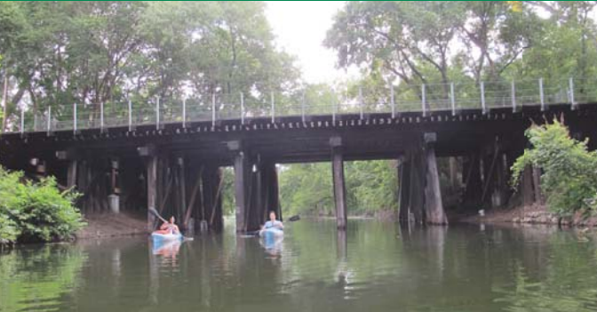
Existing Conditions | View 3
