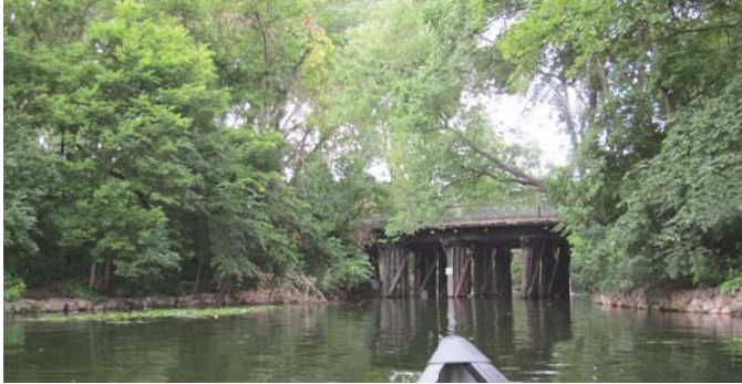
Existing Conditions | View 1
