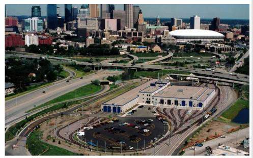
ABOVE: The operation and maintenance facility for METRO's Blue Line (formerly Hiawatha LRT) performs all the duties that will be performed at the maintenance facilities for the Green Line and Southwest LRT (Green Line extension), as well as heavier maintenance.
