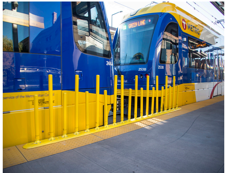
Stations include safety features such as between car bollards and tactile warning strips
