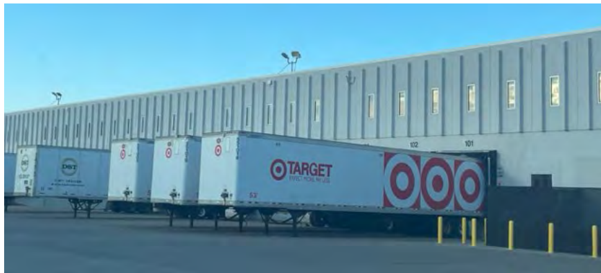
Figure: Target Sortation Facility in Minneapolis, MN
