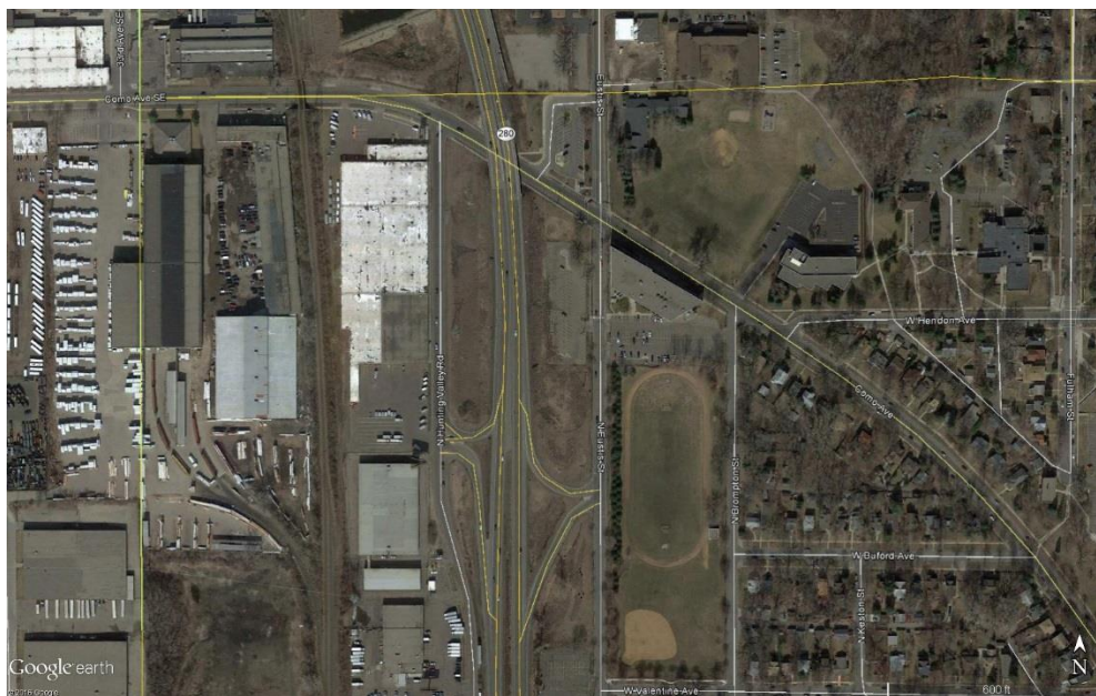
Figure 4-17: TH 280 and Como Avenue Interchange Aerial View
