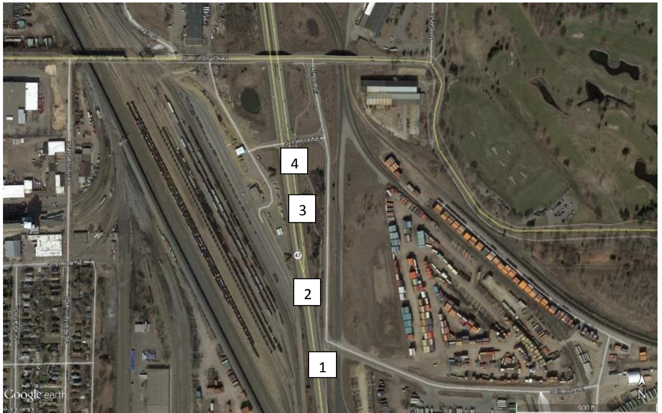
Figure 4-15: University Avenue near Intermodal Facility Aerial View
