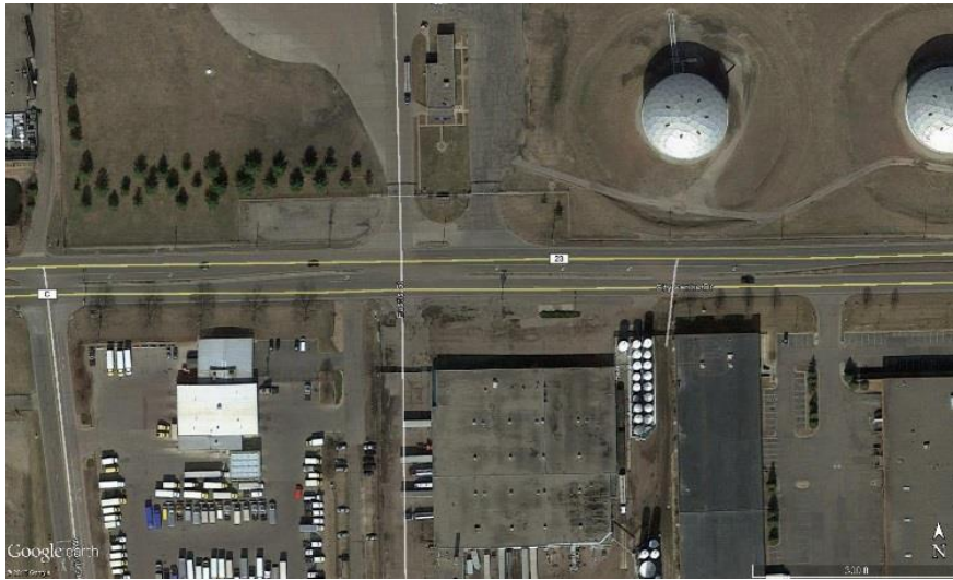
Figure 4-23: County Rd C and Petroleum Plant Aerial View
