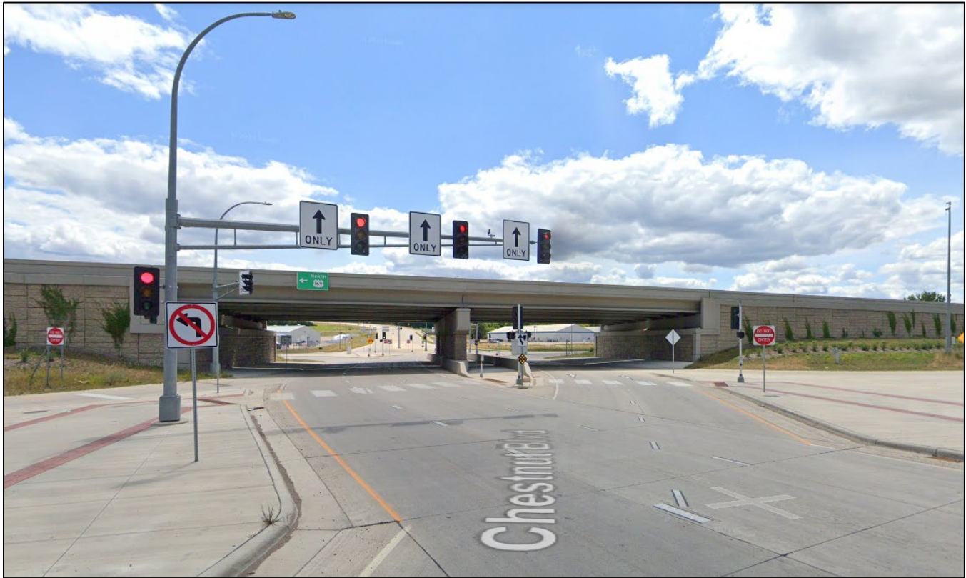
Figure 4. Highway 169 and Highway 41 grade separation in 2021 (courtesy of Google).
