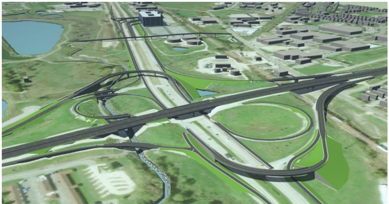
Freeway System Interchange Example
