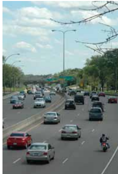
A lane in each direction was added to State Highway 100 from Excelsior Blvd. to Cedar Lake Road for approximately $7.1 million. An example of a CMSP project already implemented and benefiting travelers, the project significantly reduced crashes and resulted in relieving about 10 miles of congestion.
