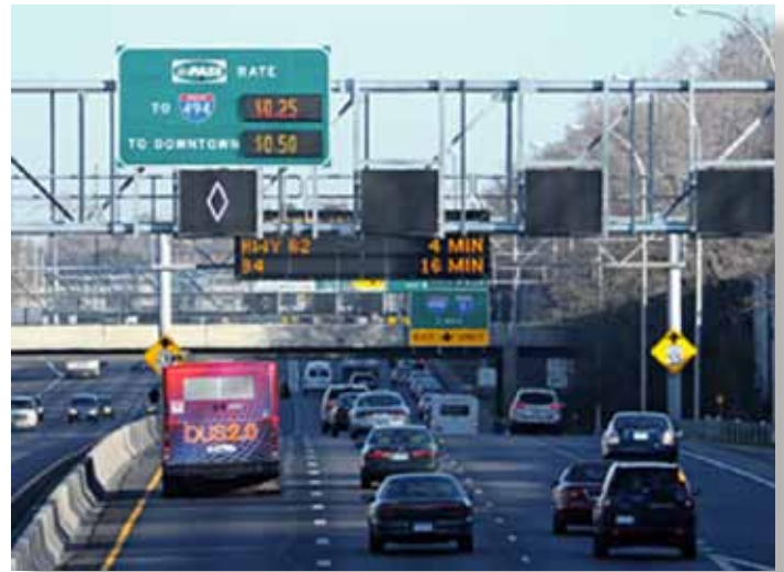
The Urban Partnership Agreement (UPA) project, that brought $133 million in federal funds for congestion relief in the I-35W corridor, shows how several different strategies can be used to address issues in one corridor. Pictured above is a MnPASS lane with motorist information signs to indicate incidents ahead.
