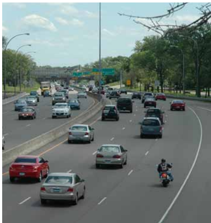
A project to construct an additional lane for a short distance on State Highway 100 in St. Louis Park (between Excelsior Blvd. and Cedar Lake Rd.) helped ease a bottleneck in the corridor.
