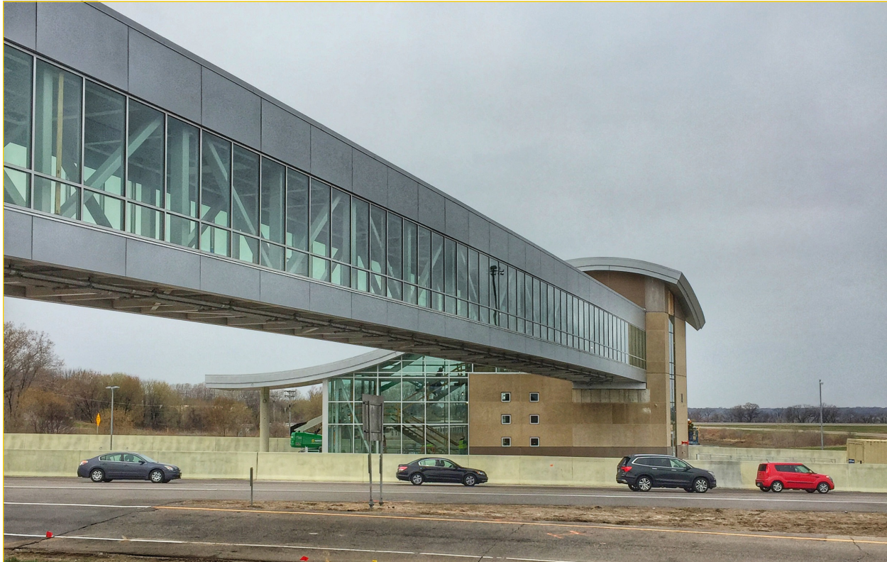
Newly Constructed Transit Station
