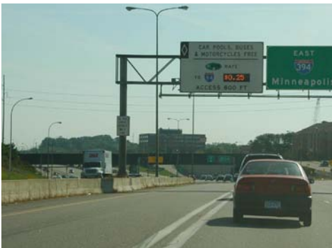
Figure 2-9: HOT lanes represent a method to add market forces to manage congestion.
