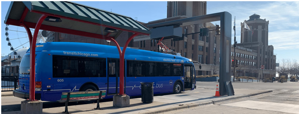
Figure 34. CTA Proterra BEB with Overhead Charger
