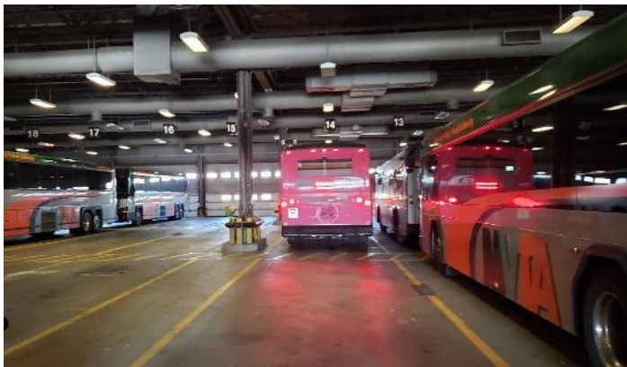
Figure 3: Enclosed bus parking / Future Charging
