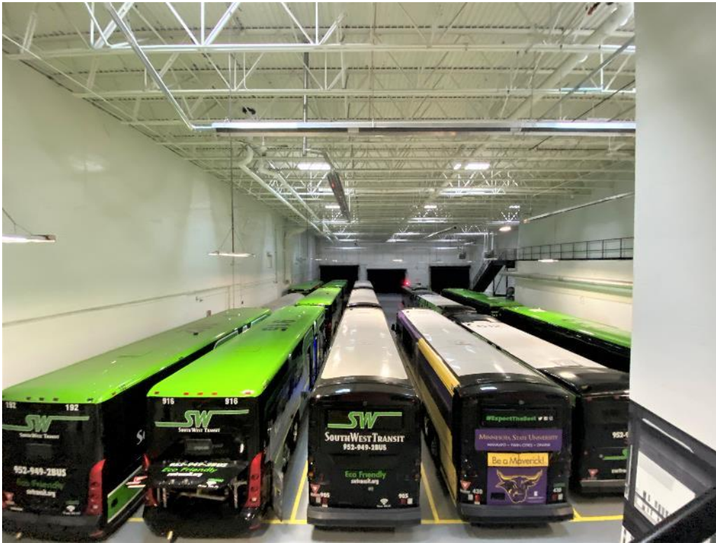
Figure 52 - View into Parking Garage B with High Ceiling & Mezzanine and Access Stair to the Right
