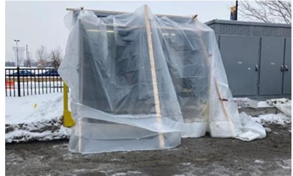
Figure 29. Temporary Charger Heating Structure
