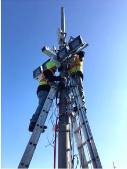
Figure 32: Illuminator and CCTV Camera
