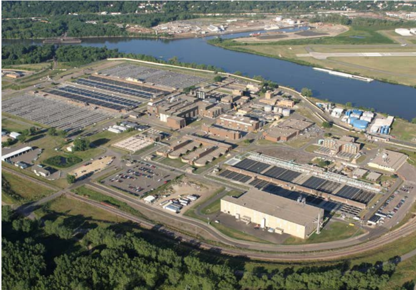
Metropolitan Wastewater Plant, St. Paul
