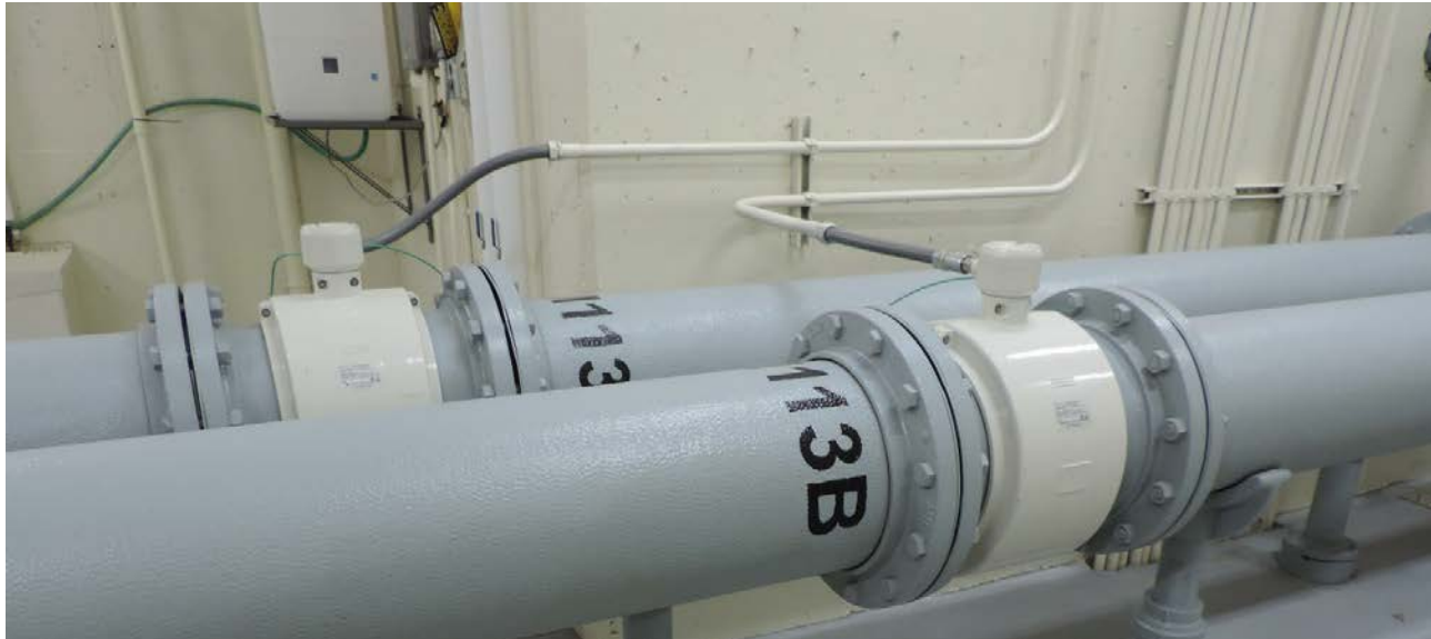
Photo of typical flow meter
