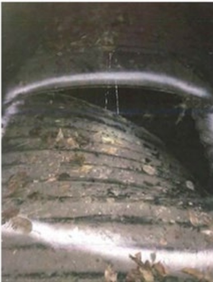
Left: Profile drawing of interceptor pipe. Right: Photo of damage to piping.
