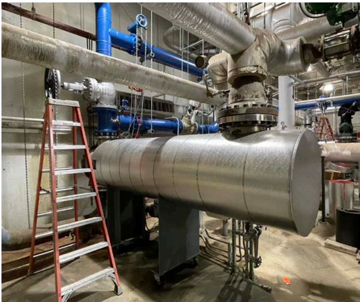
Existing Auxiliary Condenser to be Relocated
