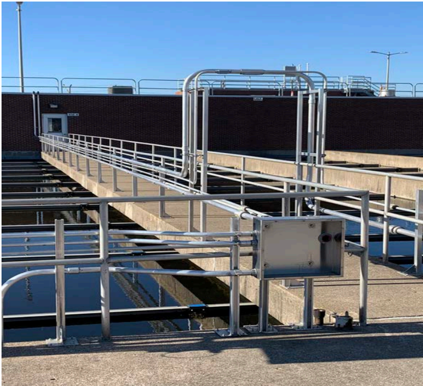
Electrical Conduit for Secondary Collector Motors
