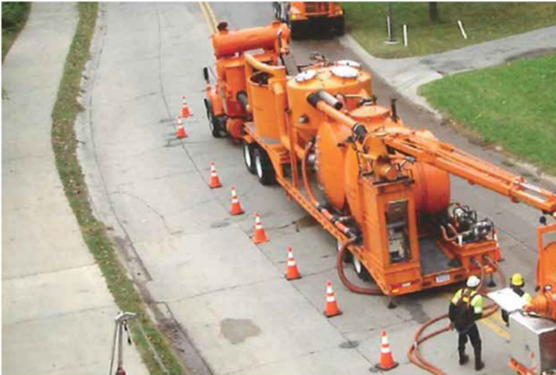
Contractor's cleaning equipment layout
