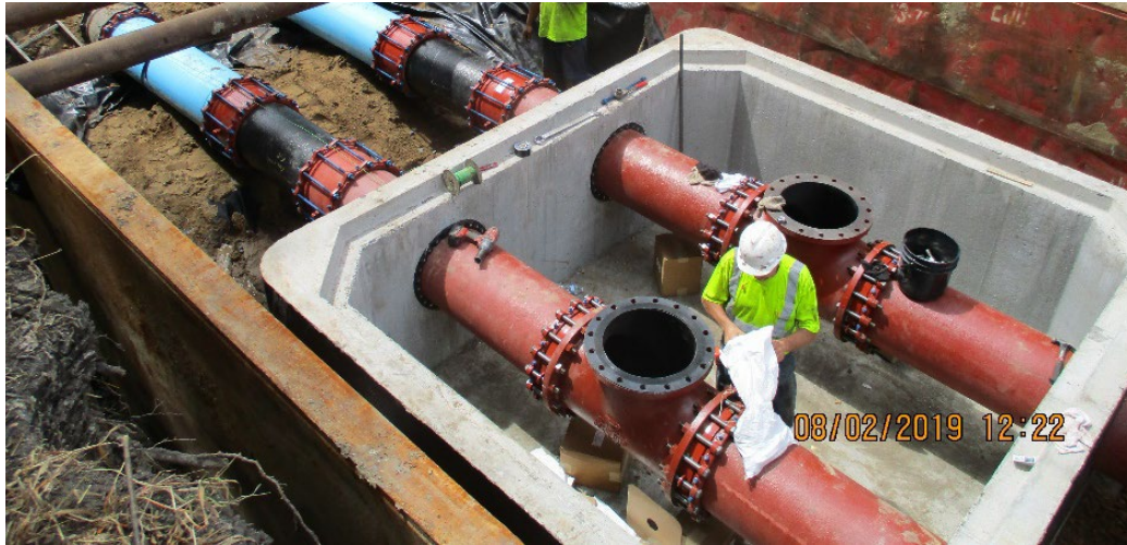
Contractor installation of 7071 Forcemain
