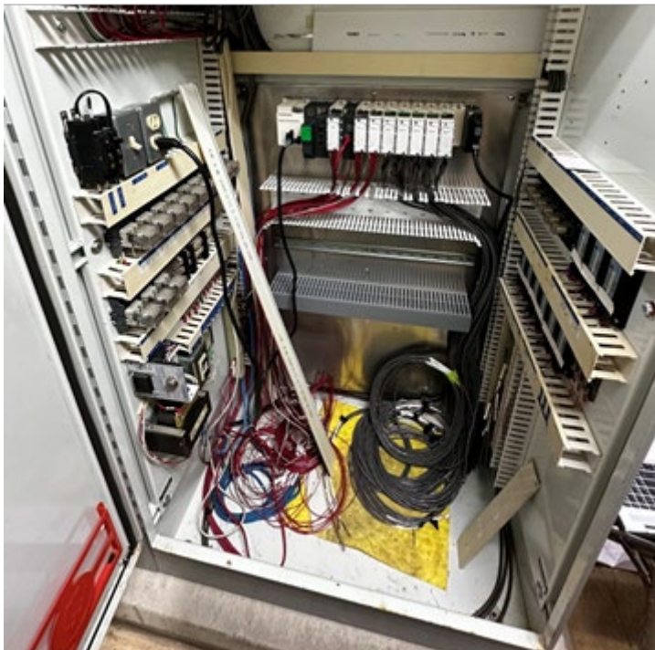
Photo taken inside a typical Programmable Logic Controller (PLC)
