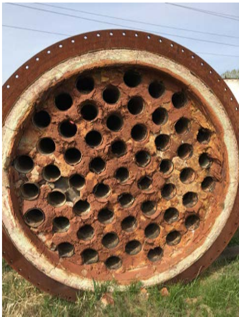
Existing Primary Heat Exchanger to be Rehabilitated
