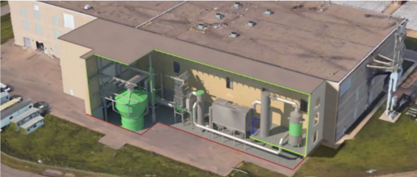
3D rendering design of future Fourth Incinerator at Metro WRRF
