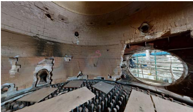
Incinerator Refractory Rehabilitation
