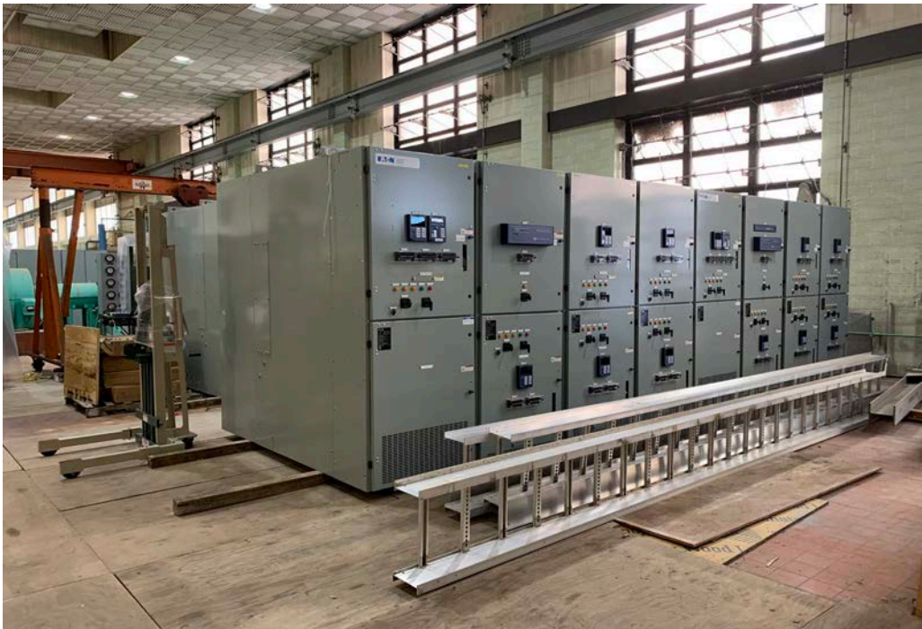
New unit substations to be installed
