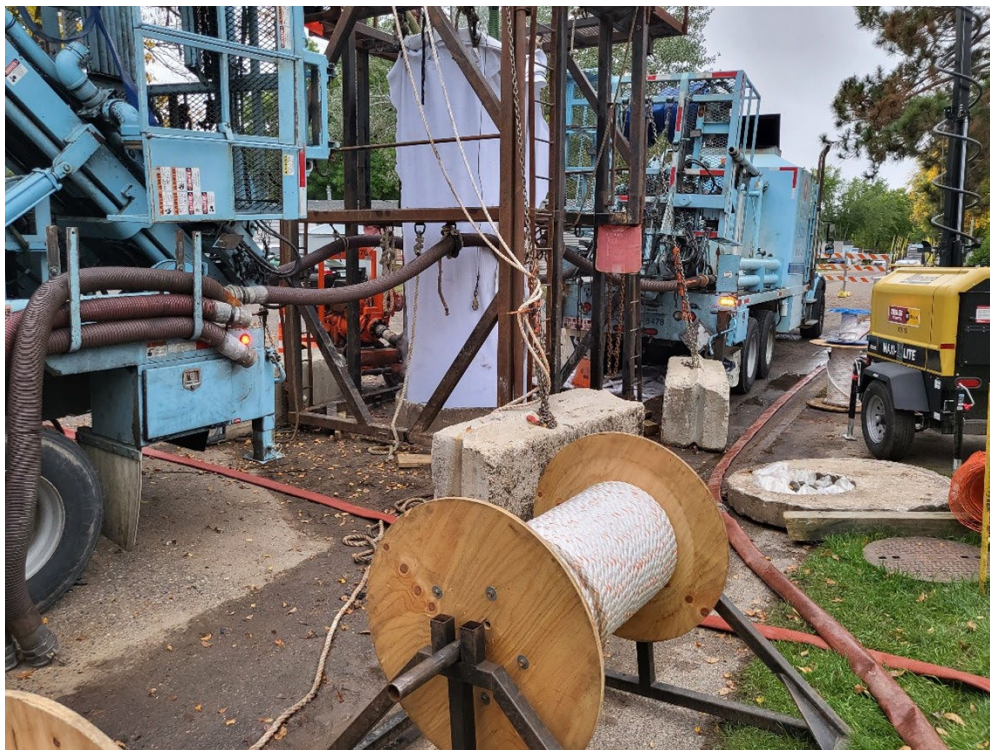
Lining work being performed on the 4-NS-525 Interceptor in Coon Rapids
