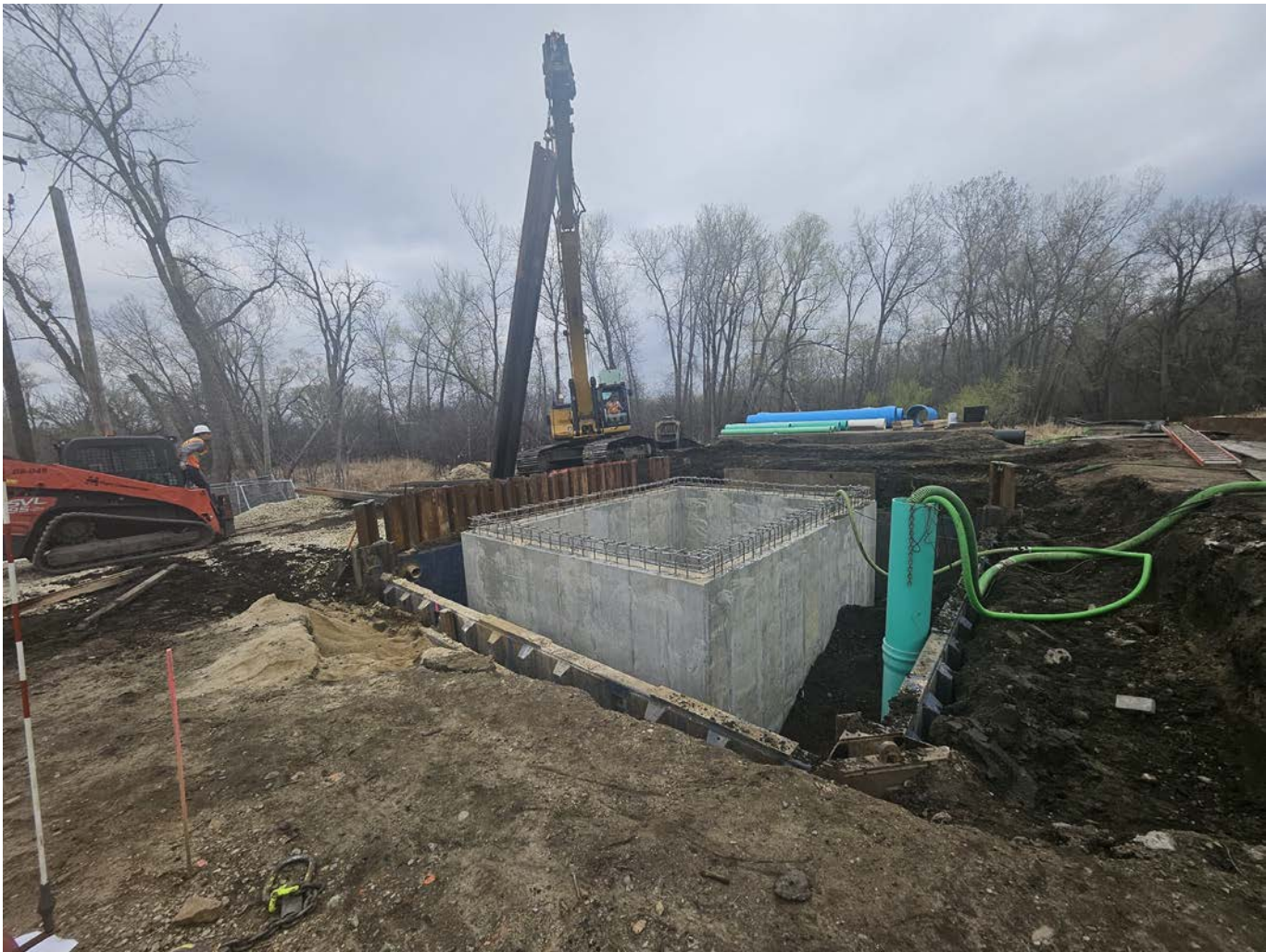
The construction of a new outfall structure for the Bloomington siphon in Eagan
