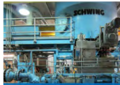
Cake Pumping Modifications
