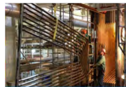
Waste Heat Boiler Tube Replacement
