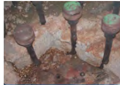
Fluid Bed Incinerator Air Distribution
