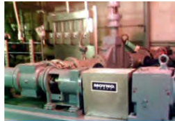
Sludge Storage Pumping Improvements
