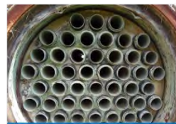
Primary Heat Exchanger Renewal
