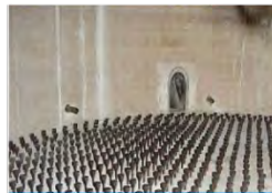
Fluid Bed Incinerator Rehabilitation
