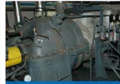
Turbine Generator Improvements
