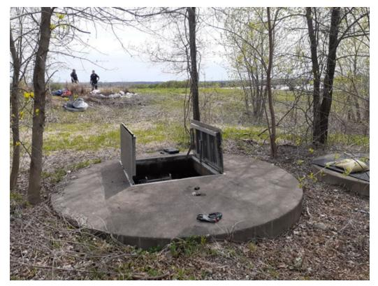
Photo of typical maintenance access structure
