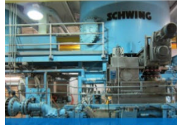
Cake Pumping Modifications
