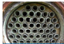
Primary Heat Exchanger Renewal
