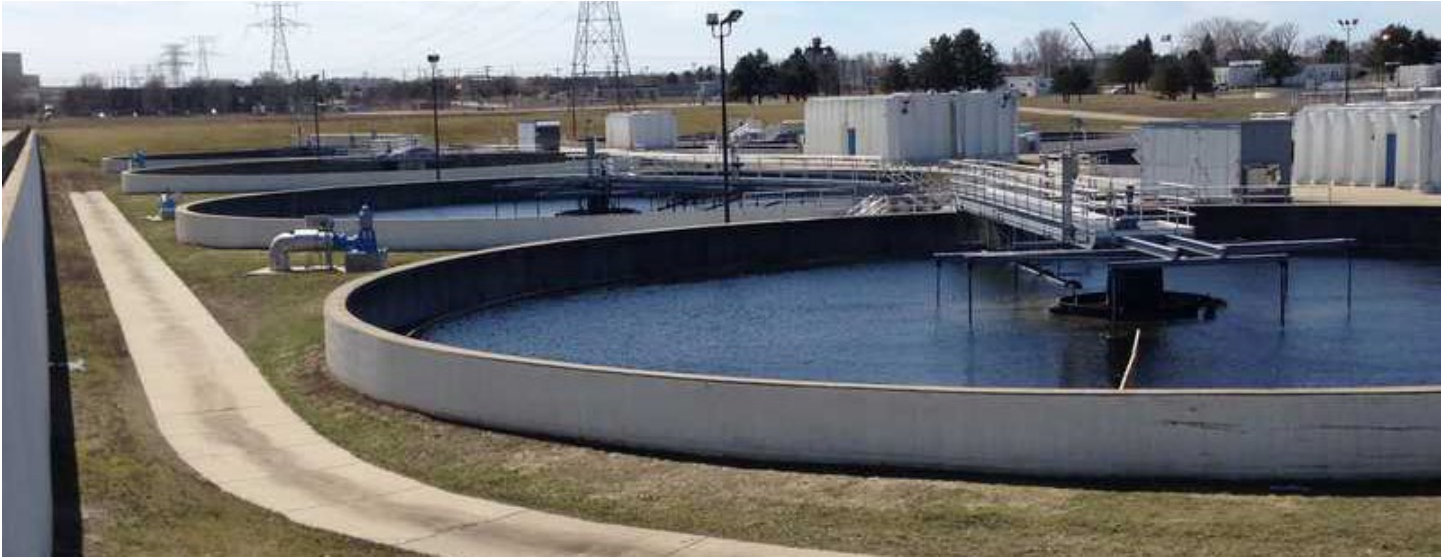
Blue Lake Wastewater Treatment Plant (WWTP)
