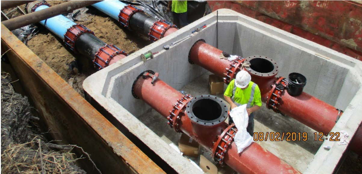
Contractor installation of 7071 Forcemain
