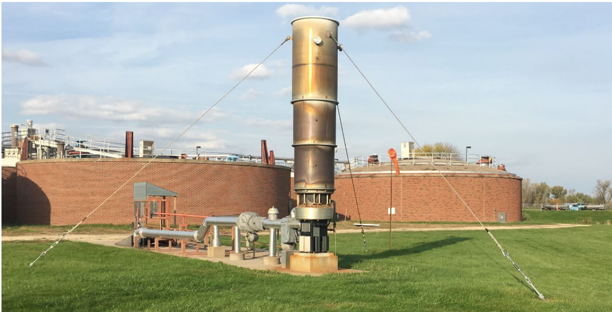
Biogas flare and Digesters 4 and 5 at Empire WRRF
