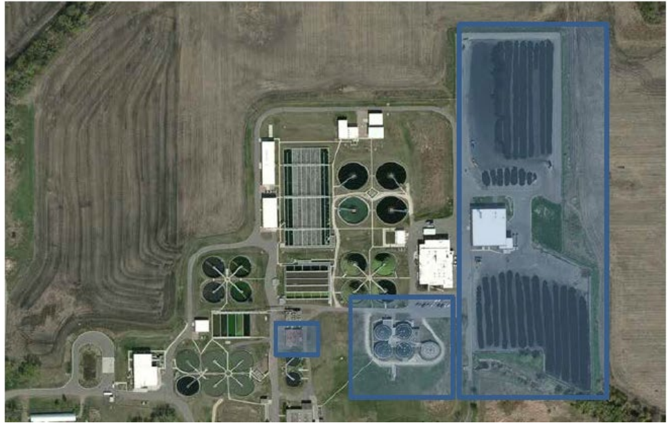
Aerial view of Empire Wastewater Treatment Plant (WWTP)
