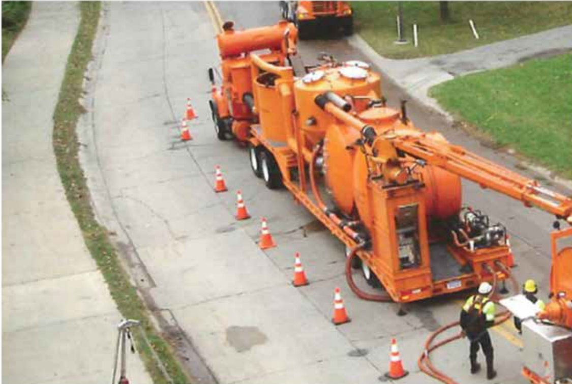
Contractor's cleaning equipment layout
