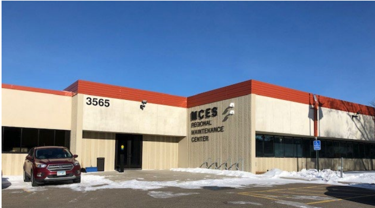
Regional Maintenance Facility (RMF)
