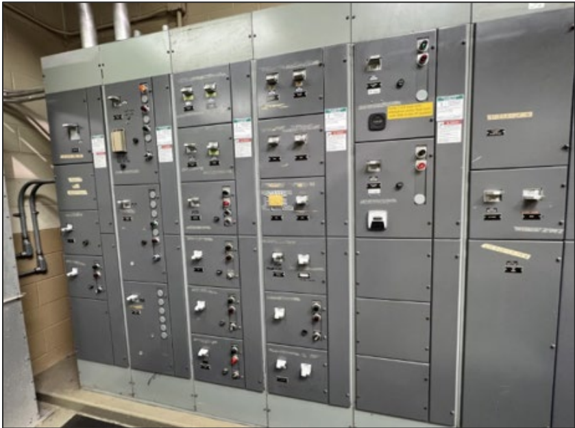
Existing motor control centers (MCCs) at lift station L31.
