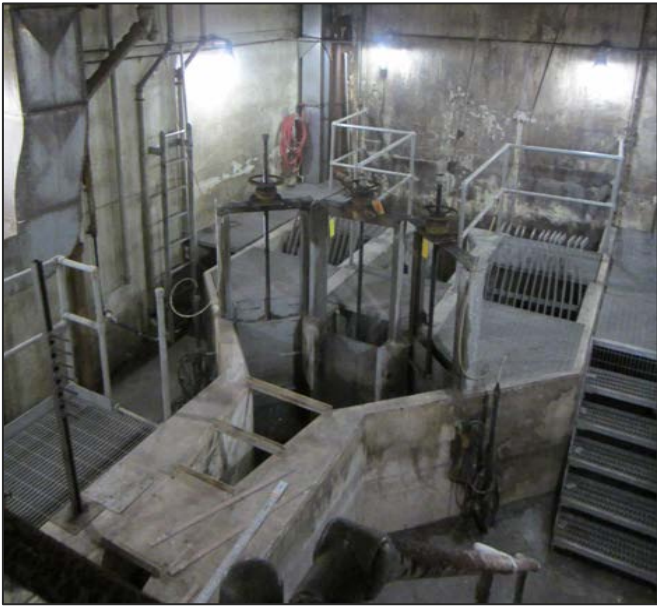
Lift Station L35 wet well
