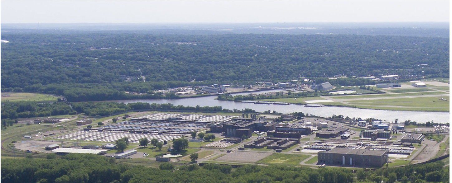
Metropolitan Wastewater Treatment Plant (WWTP)
