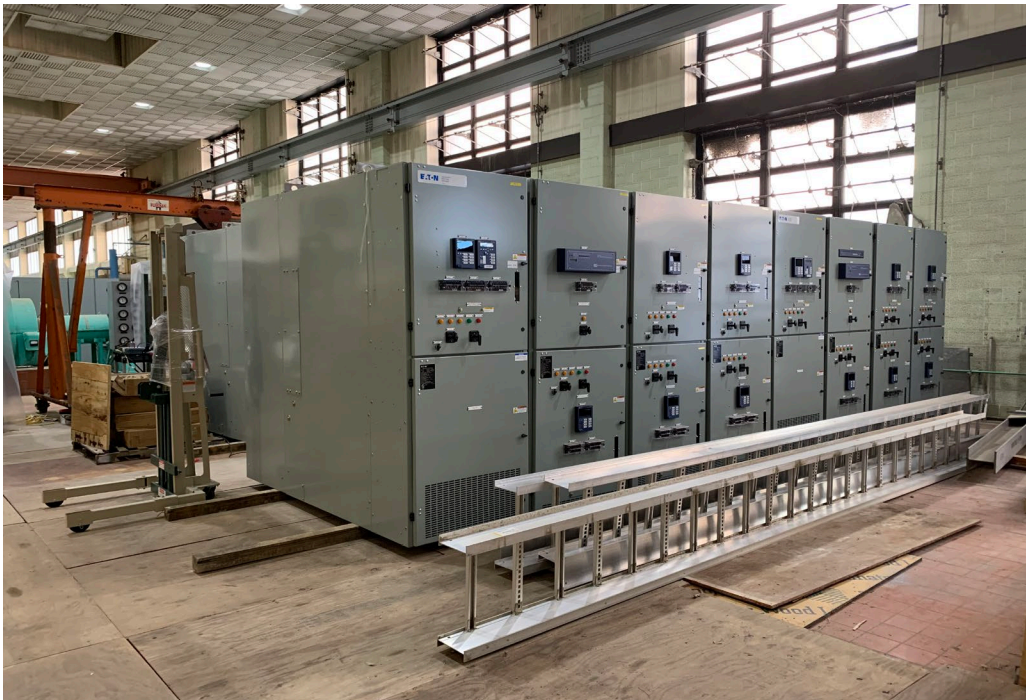
New unit substations to be installed
