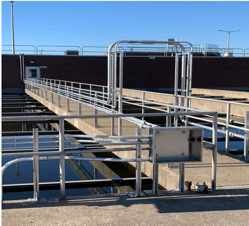
Electrical Conduit for Secondary Collector Motors
