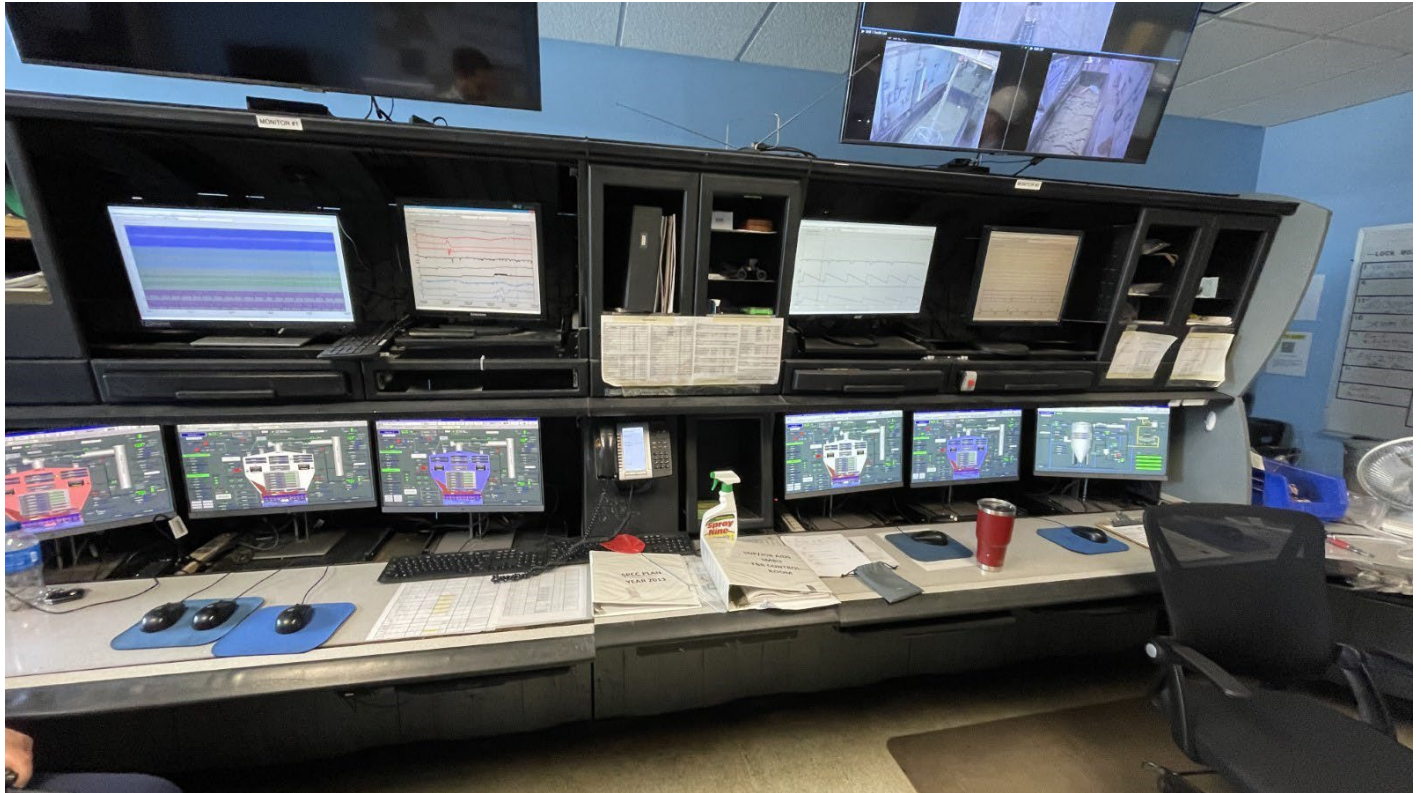
Existing Metro Plant Solids Management Building Control Room built in 2004.
