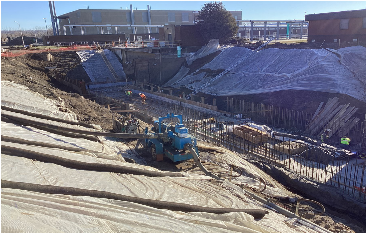
Construction of the new tunnel from EPR to Services Building
