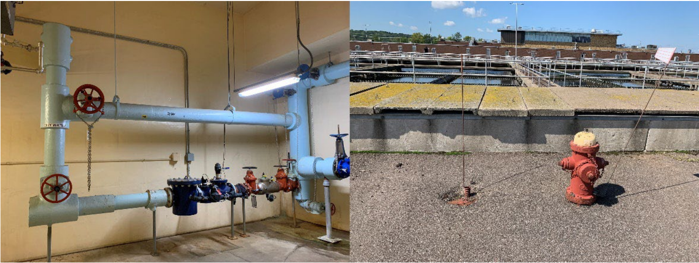
Left: One of two water metering stations which is located near East Primary. Right: City water hydrant and isolation valve at final sedimentation tanks.
