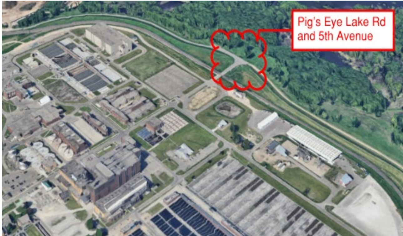
Flood control measure location at the Metro WWTP at Pig's Eye Lake Road and 5 th Avenue
