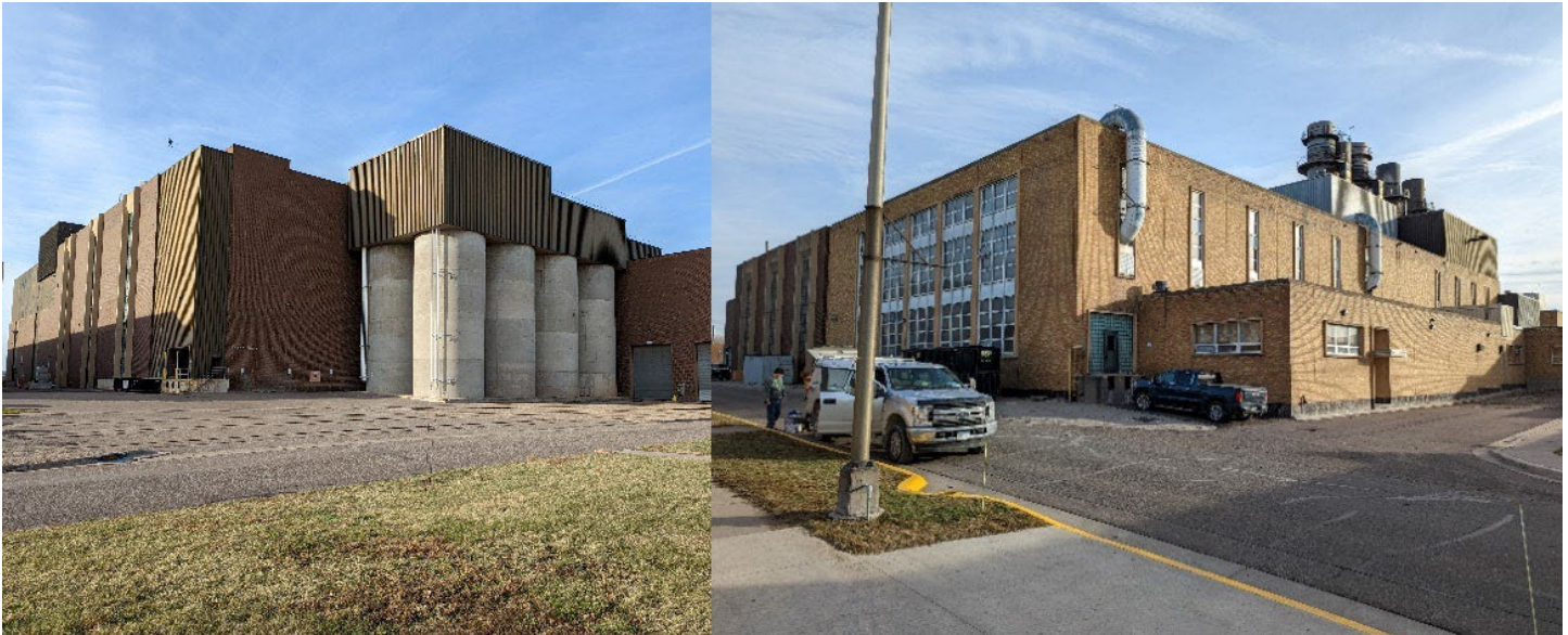
Left: 408 Building looking west. Right: F&I #2 building looking east.
