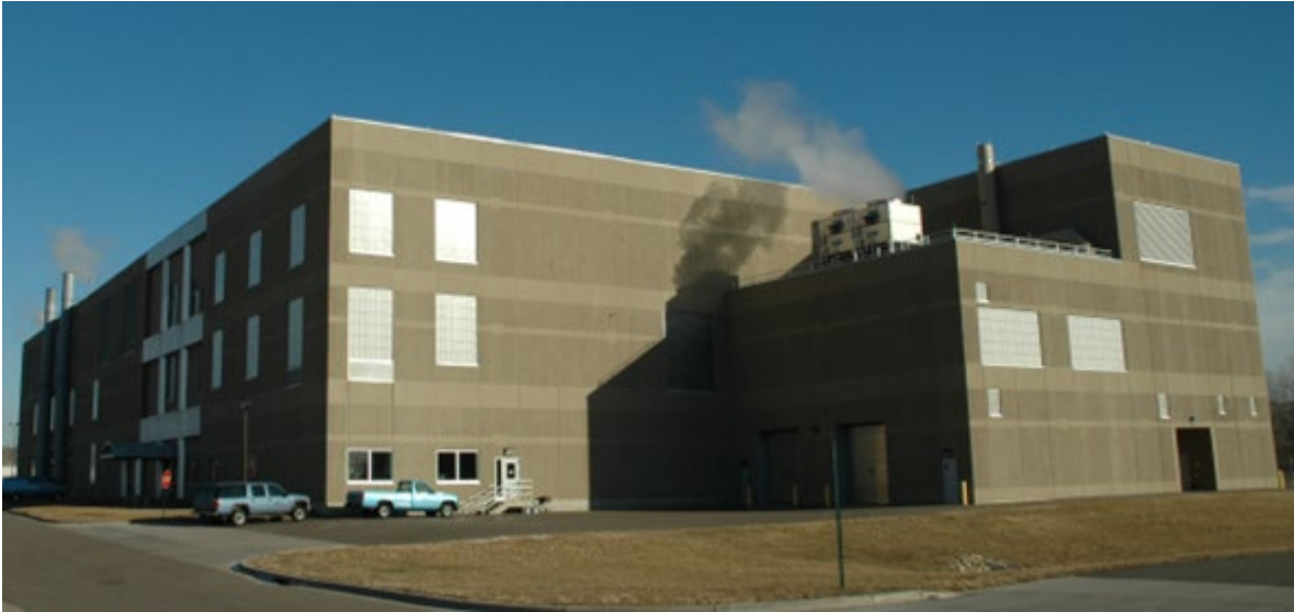
Metropolitan Wastewater Treatment Plant (WWTP) Solids Management Building (SMB)
