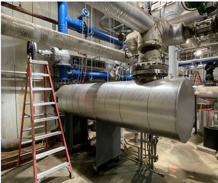
Existing Auxiliary Condenser to be Relocated
