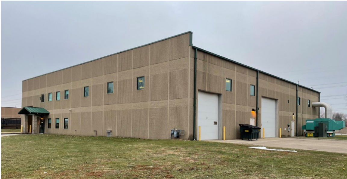
Fridley Liquid Waste Receiving Facility
