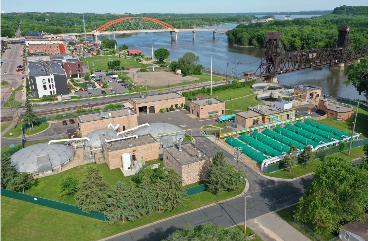
Aerial view of existing Hastings Water Resource Recovery Facility
