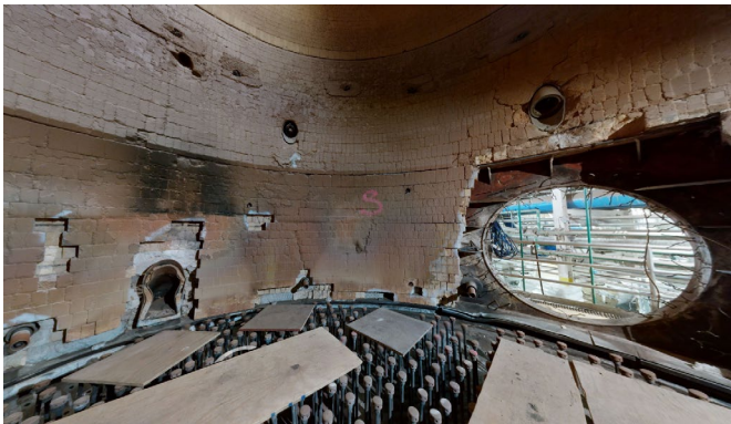
Incinerator Refractory Rehabilitation
