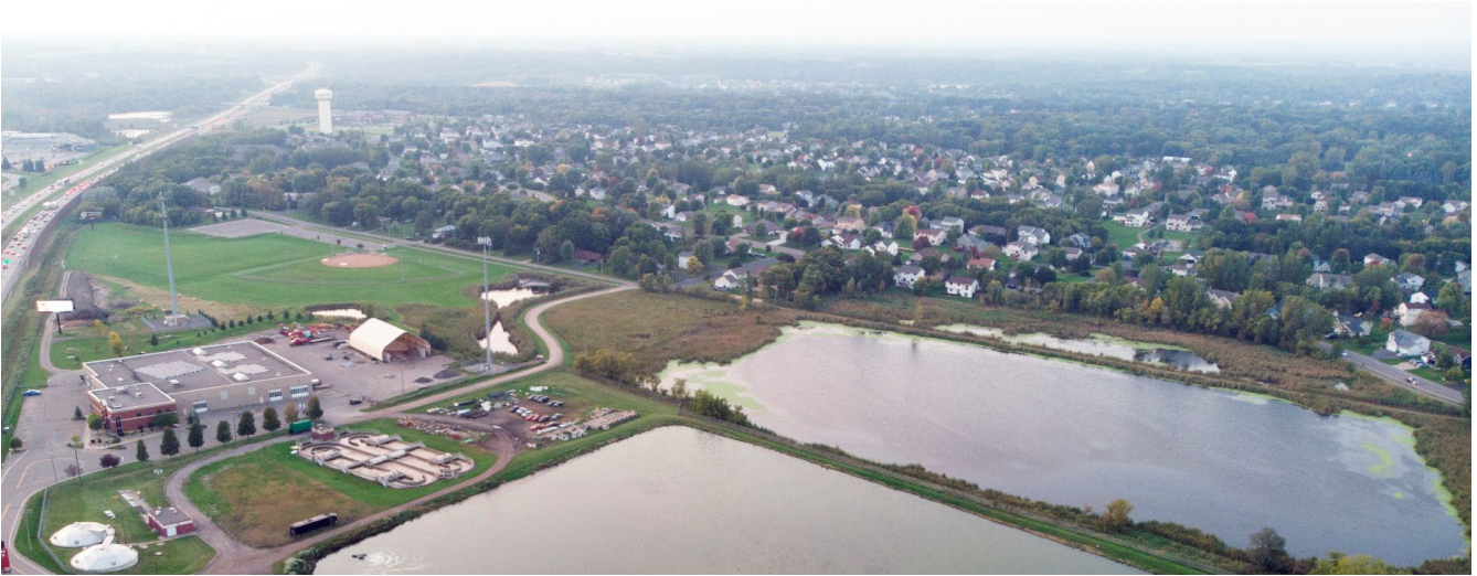
Aerial view of the Rogers Wastewater Treatment Facility acquired by ES in 2018
