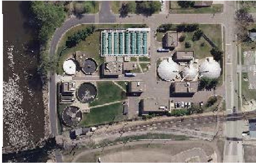
Aerial View of Hastings WWTP
