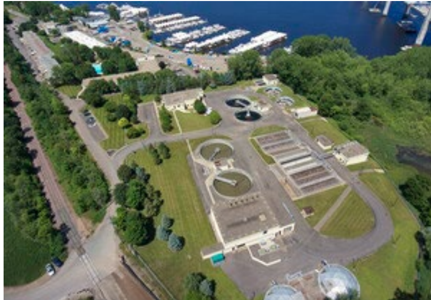
Aerial photo of St. Croix Valley WWTP
