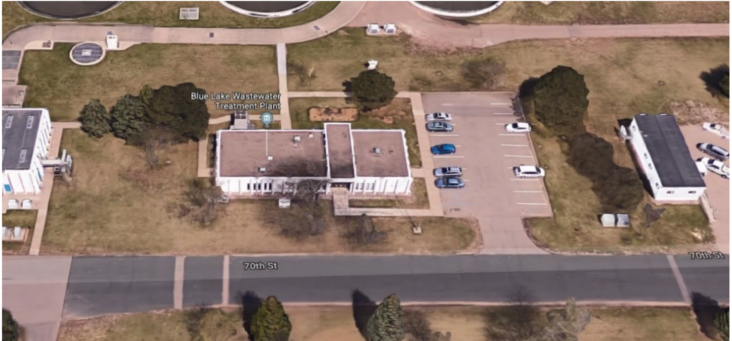
Blue Lake WWTP Administration Building
