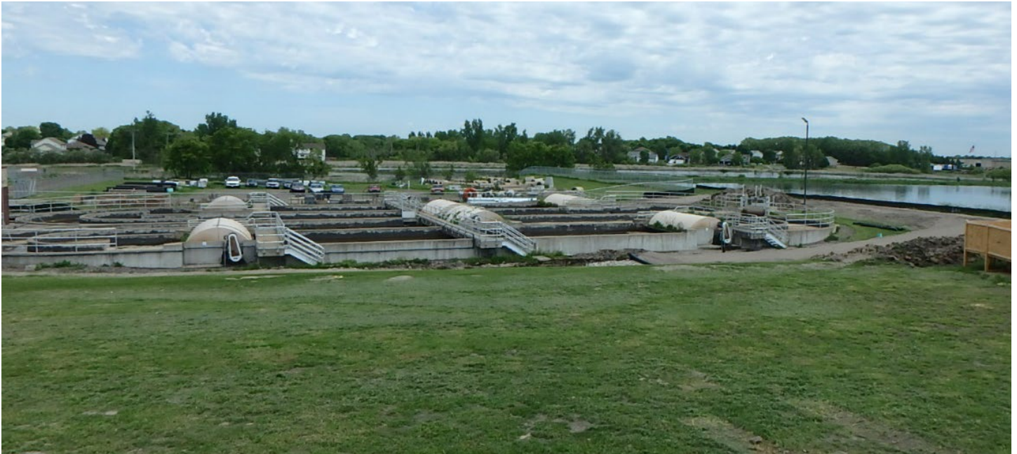
Photo of Rogers WWTF
