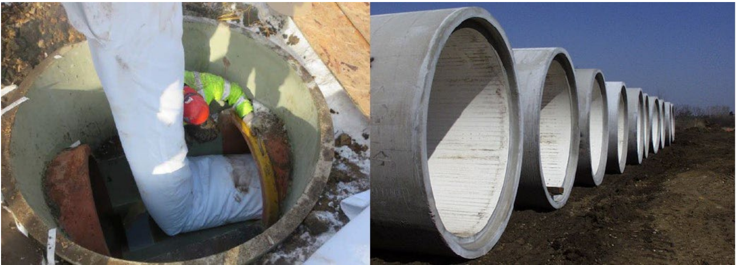
Left: Cured-in-Place (CIP) pipe liner being installed through a maintenance hole. Right: Large-diameter interceptor sewer pipe segments ready for installation.
