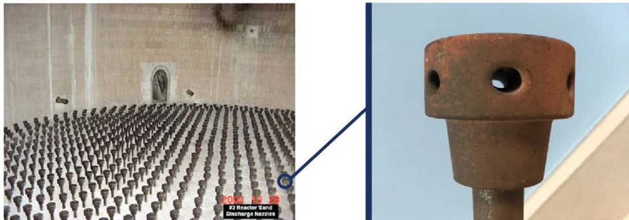
Photo 2. 1,339 tuyeres, which are 1-inch-diameter pipes with bubble caps, deliver combustion and fluidizing air to the incinerator
