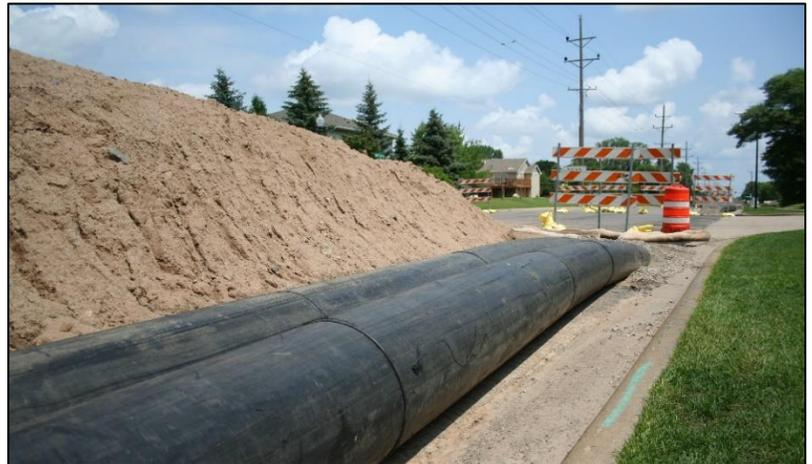
*MCES crews bury temporary wastewater conveyance pipes at intersections to maintain traffic access during sewer work*
