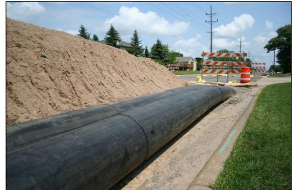
Typical view of temporary wastewater conveyance pipes
